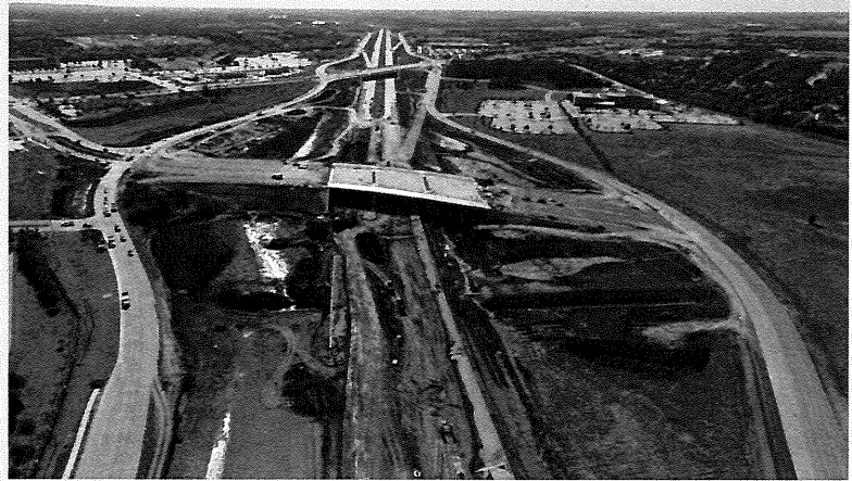
Nov. 2017 - Holland Road and Broad Street bridges over future SH 360
