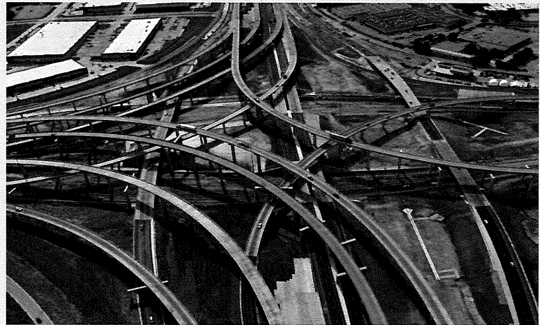
Nov. 2017 - I-35W/820 Interchange Looking South
