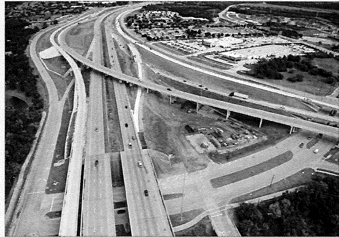
SH 121/360 interchange construction
