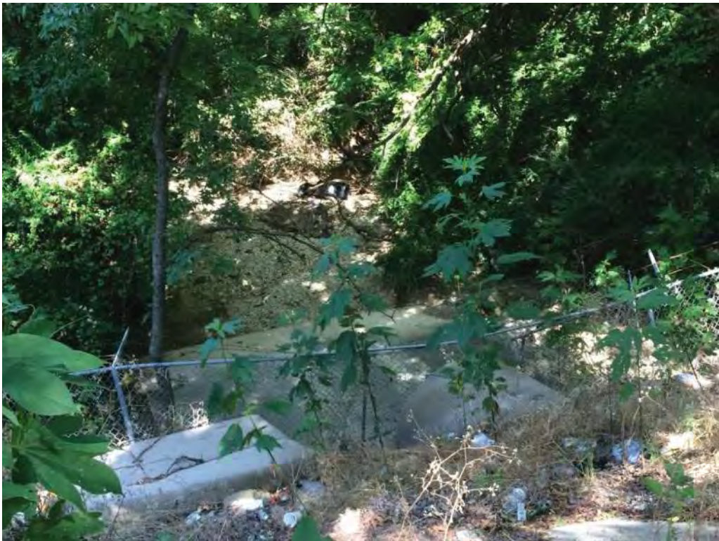
Culvert Outfall at Belle Avenue
