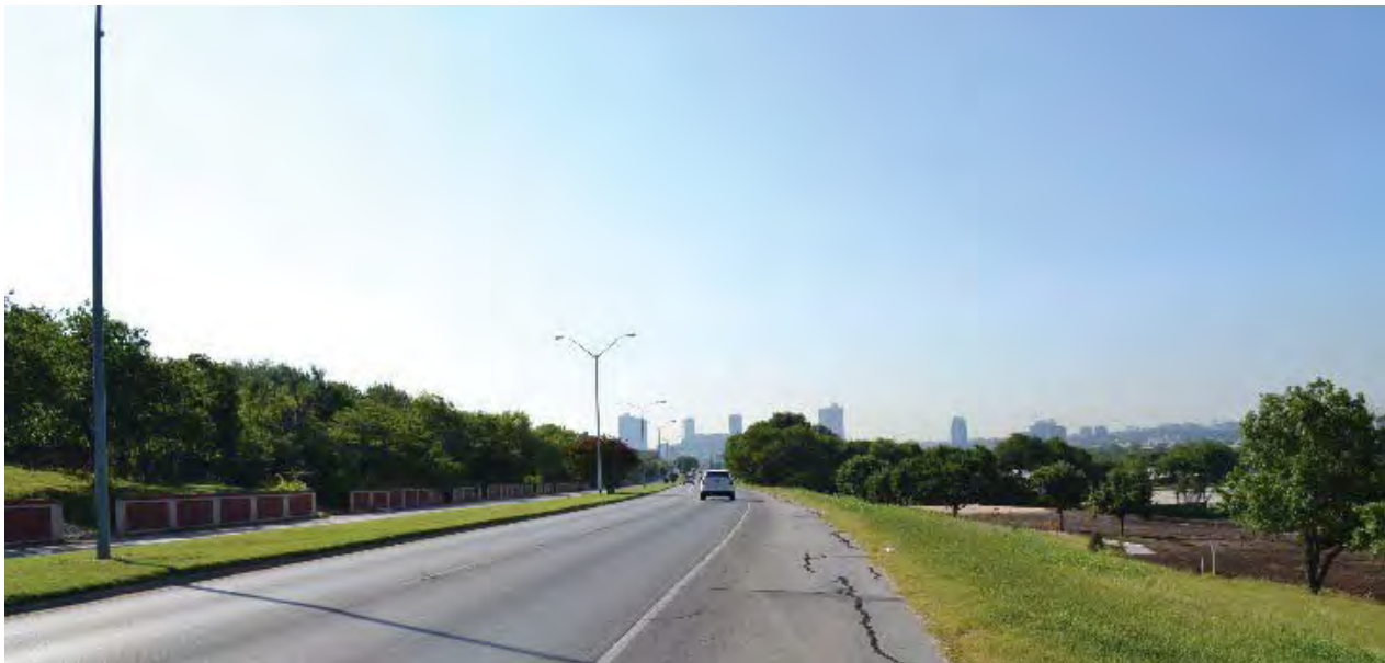
Figure 9. East Perspective Near SH 199 and 21 st Street Intersection and Rockwood Golf Course
