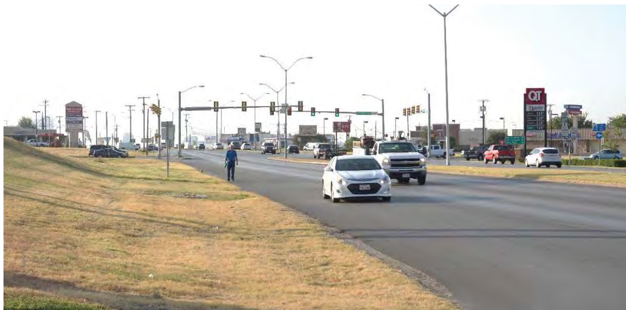
Figure 11. Pedestrian Utilizing Roadway Shoulder West of SH 199 and SH 183 Intersection
