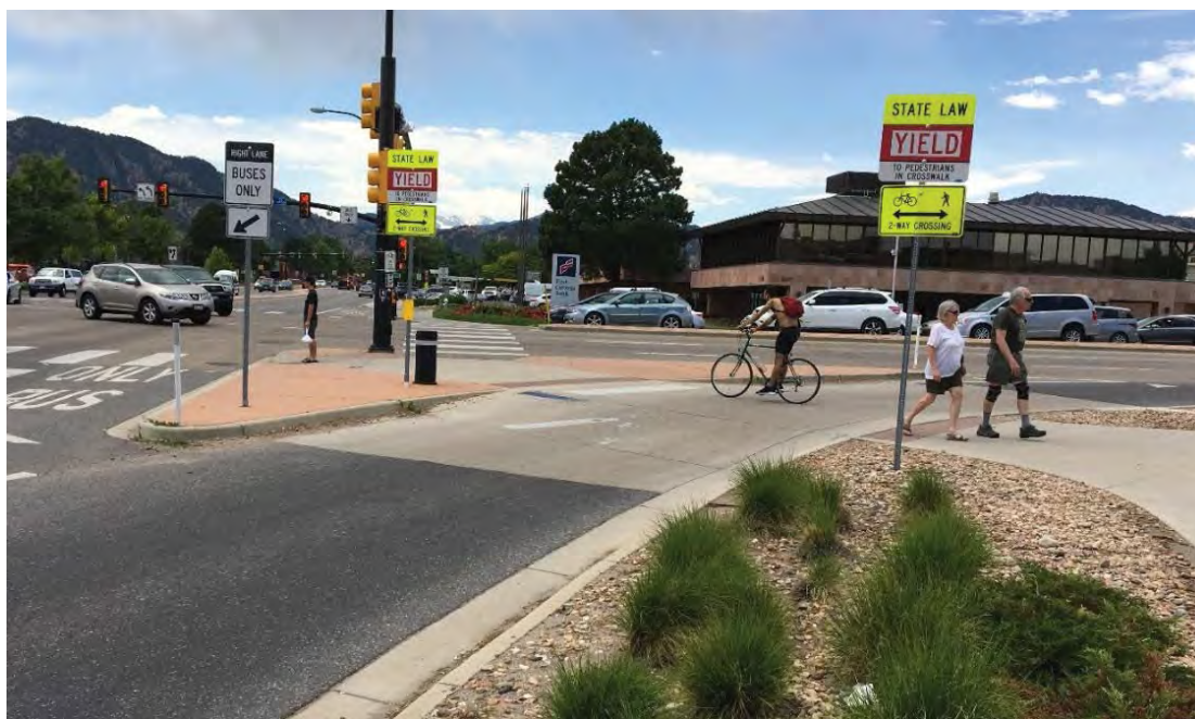
Figure 19. Perspective View of Raised Crosswalk at Right Turn Lane in Boulder, Colorado
