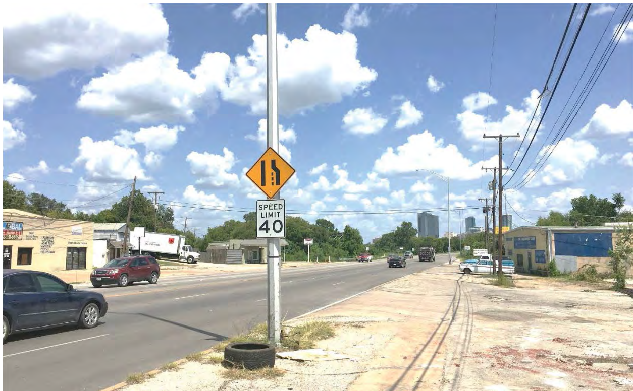
Figure 3. East Perspective of Overhead Utilities East of University Drive
