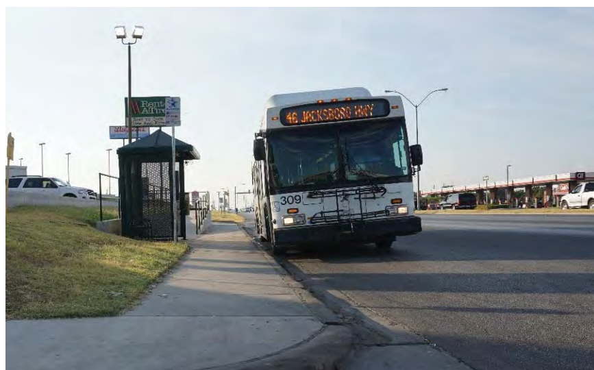
Figure 3. Existing Bus Shelter and Pull Out West of SH 199 and SH 183 Intersection at Town and Country Center
