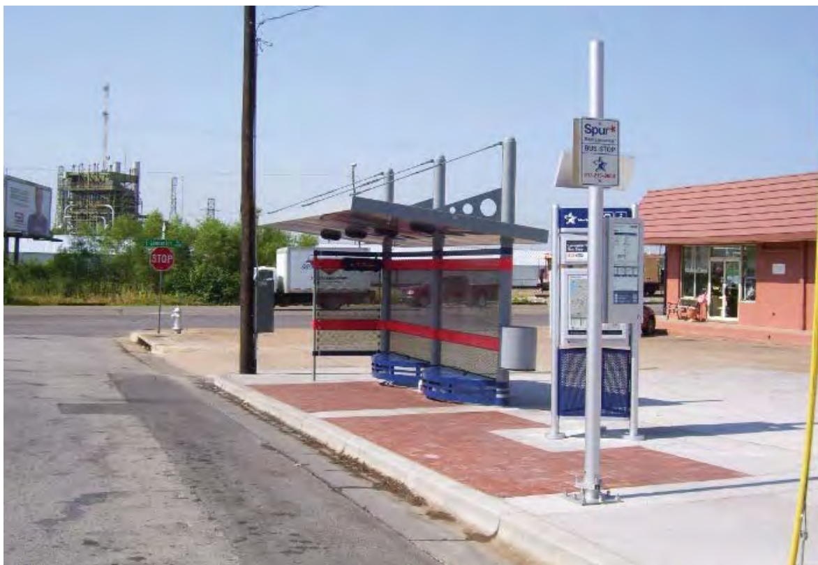
Figure 8. Enhanced Bus Shelter along Lancaster Avenue Bus Route
