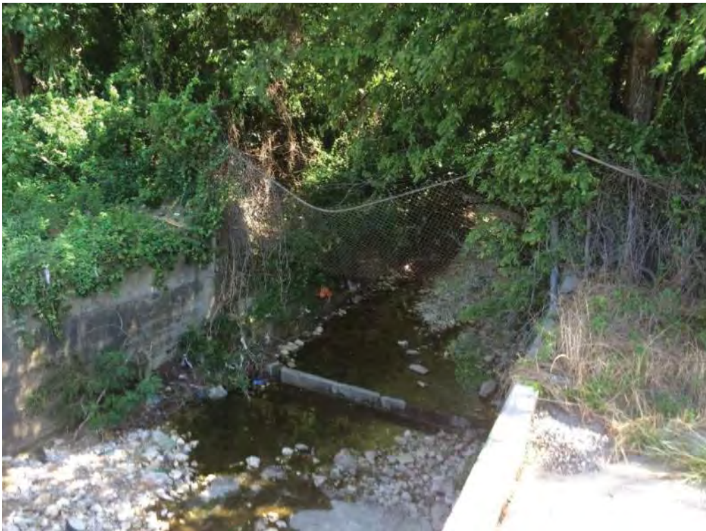
Unnamed Tributary to Stream WF-5
