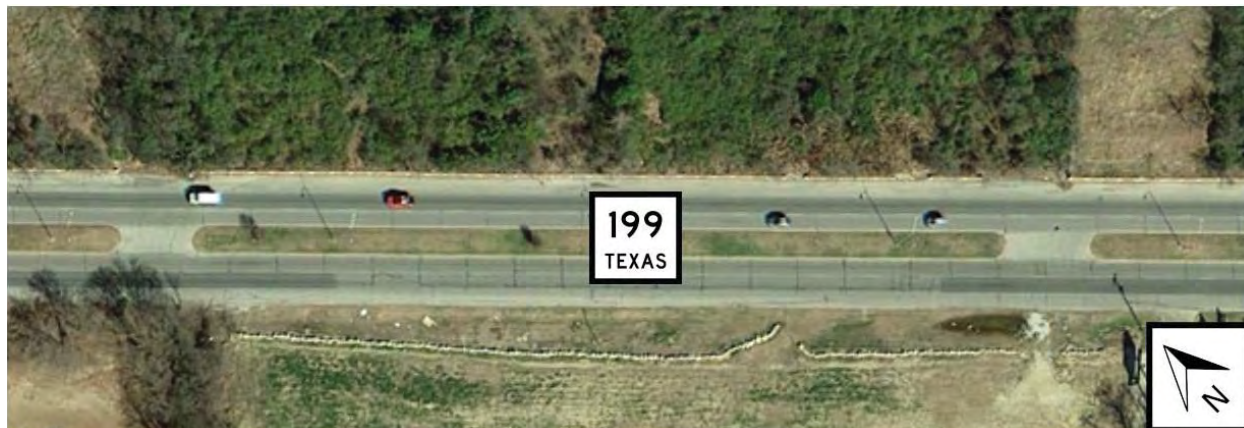
Figure 2. Existing SH 199 Median Openings Unassociated with Cross Streets or Driveways
