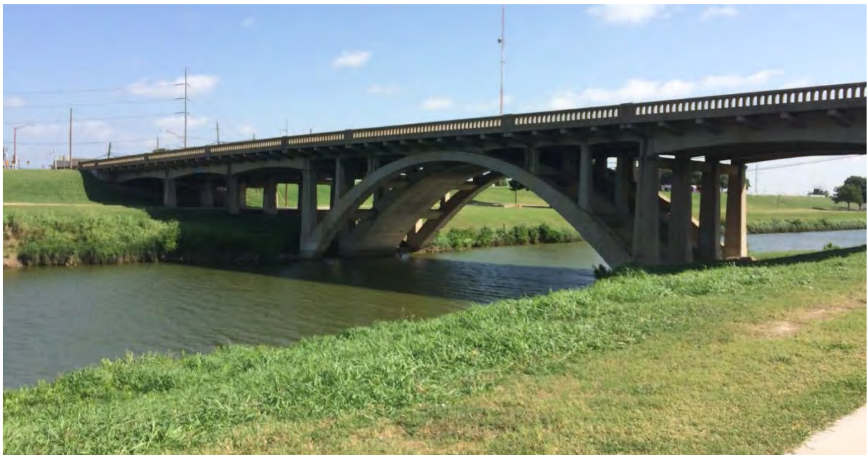
Figure 7. Photograph of Henderson Street Bridge Looking East Along Trinity River
