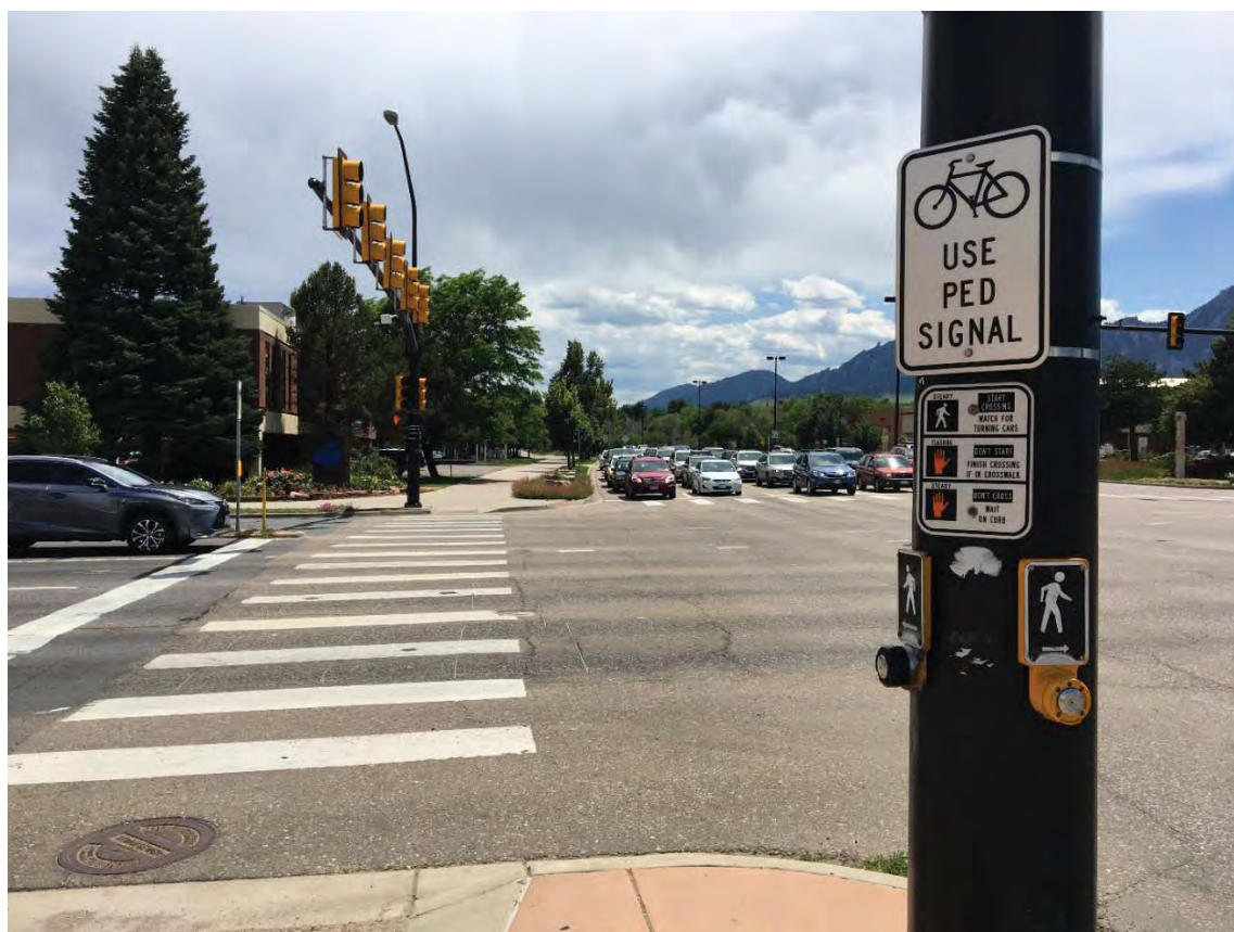
Figure 12. Bicycles Use Ped Signal Sign (R9-5) Installed with Pushbutton
