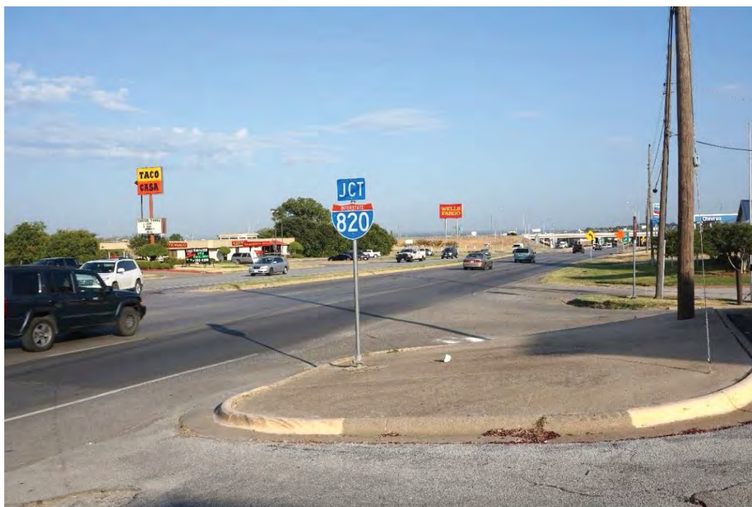
Figure 1. Typical Character Zone 1 Commercial Frontage
