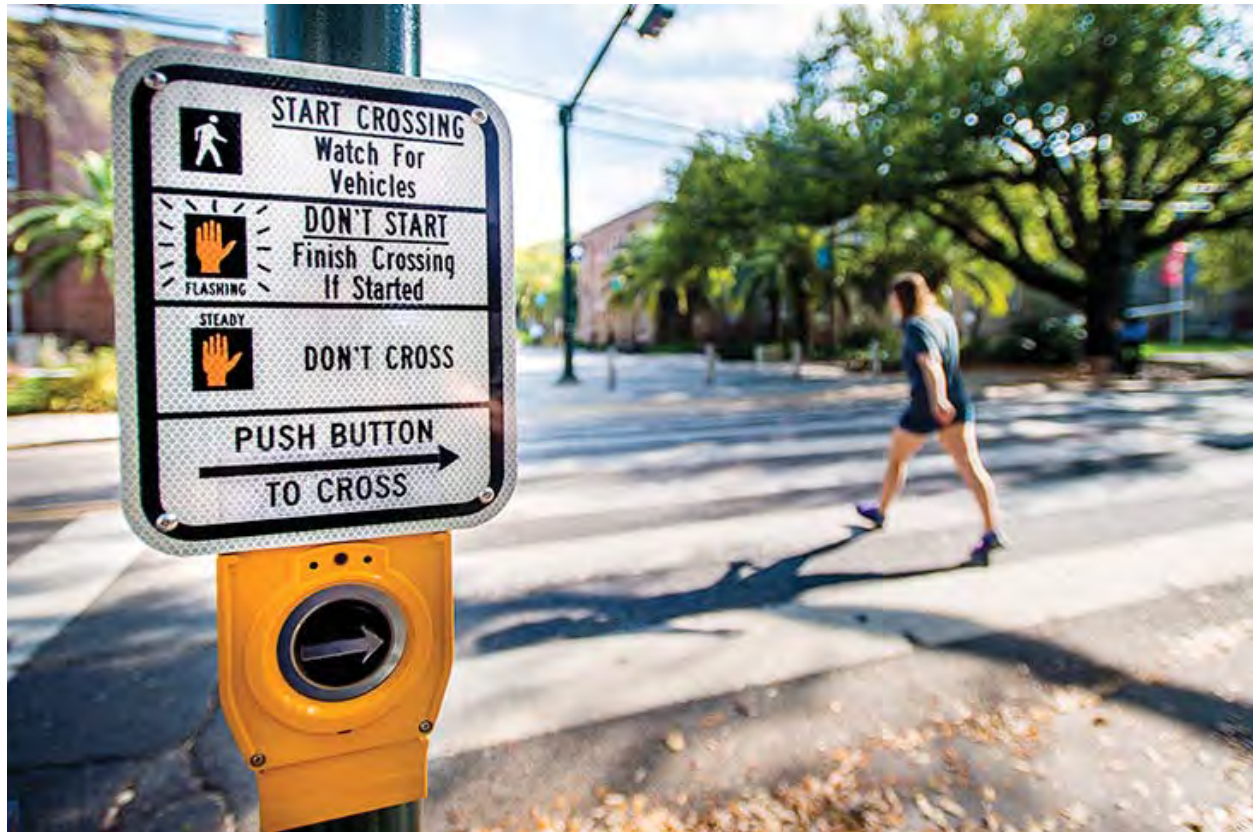
Figure 15. Accessible Pedestrian Signal Pushbutton Assembly
