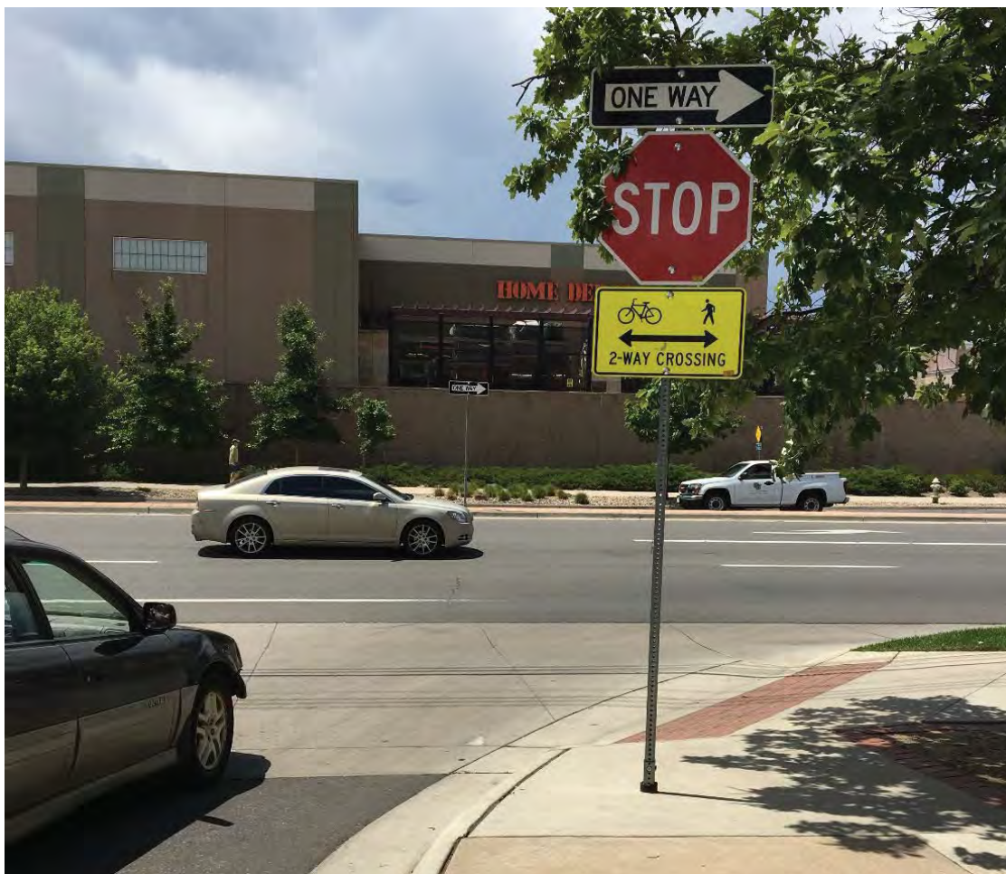
Figure 28. Signage for Two-Way Bicycle and Pedestrian Traffic at Driveway
