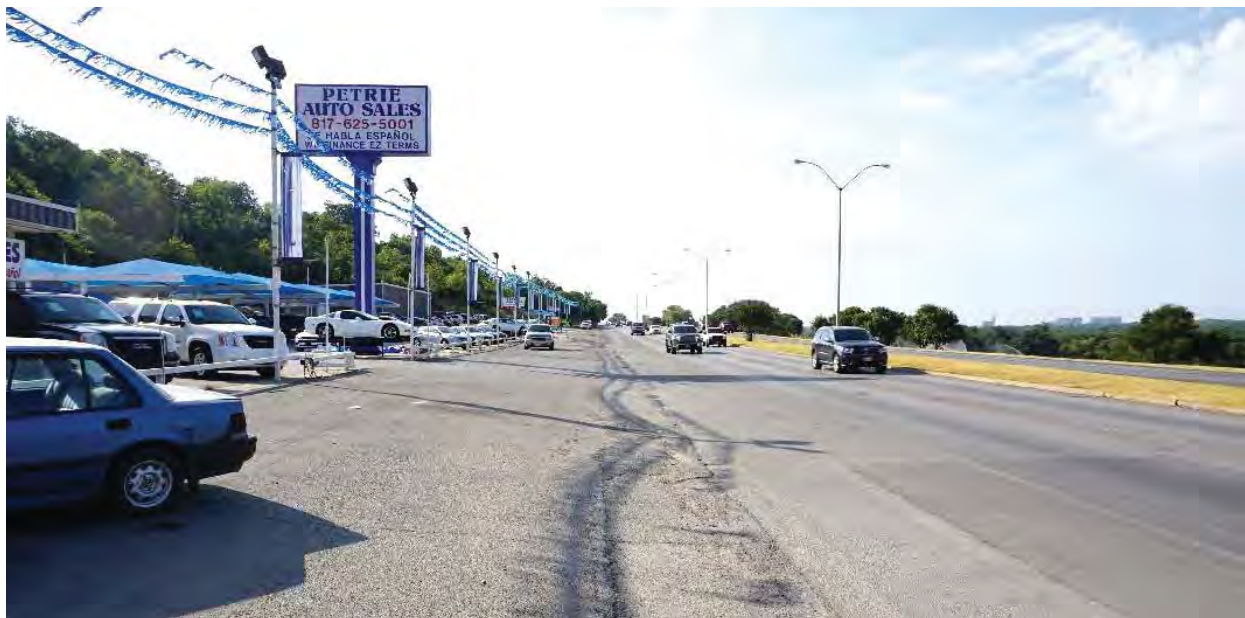
Figure 10. Paved Driveway and Shoulder East of SH 199 and 21st Street Intersection
