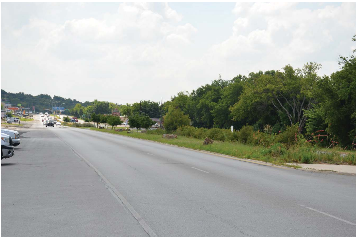
Figure 1. Landscape Median Between Roberts Cut Off Road and Skyline Drive
