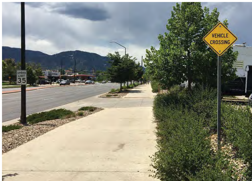
Figure 31. Signage to Warn People Walking and Biking on Enhanced Sidewalk of Potential Cross Traffic at Driveway
