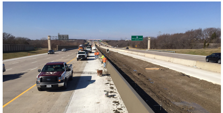
Newly constructed concrete traffic barrier for PGBT fourth lane.
