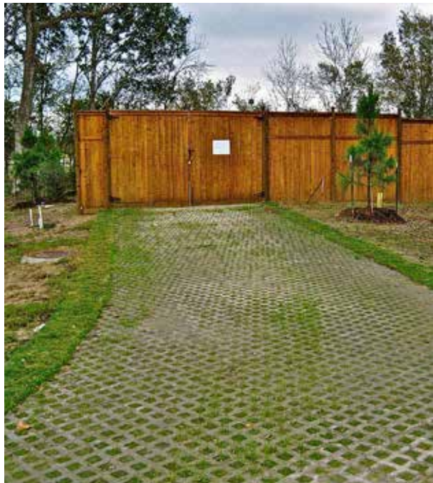
Modular Porous Paver Systems: Cliff Tuttle park, Houston, Texas (top); Houston, Texas (bottom).
