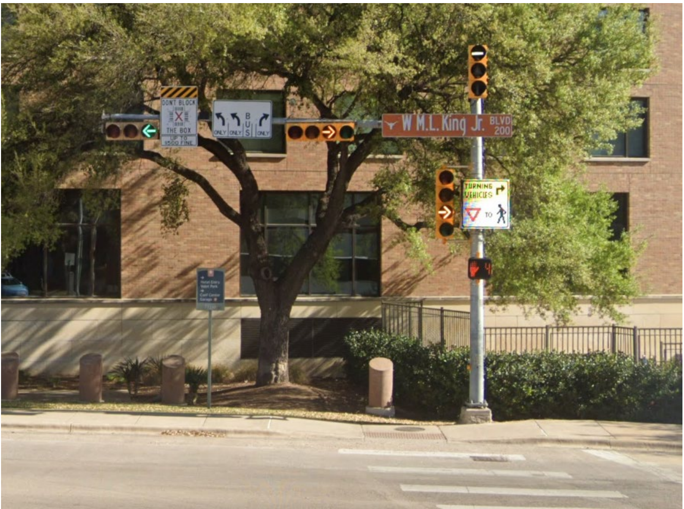
Figure 18: Example of Flashing Yellow Arrow for pedestrian conflicts ( Google Street View ). Note that Austin frequently uses dynamic ITS signs for these treatments, and the sign appearing here as Turning Vehicles Yield to Pedestrians (R10-15) is one of them.
