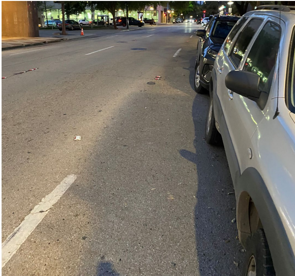
Figure 5: Pavement markings (lane skips)
