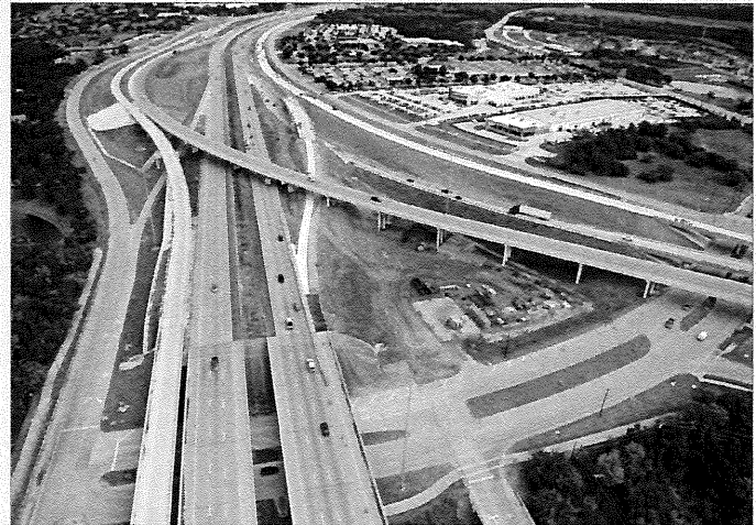
SH 121/360 interchange construction
