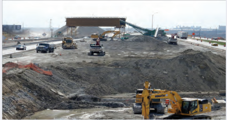
March 2017 - I-35W construction at 28th Street
