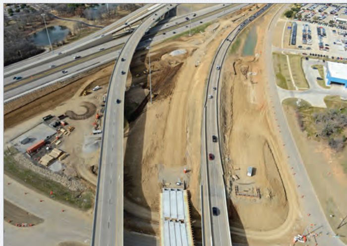
SH 121/360 interchange construction
