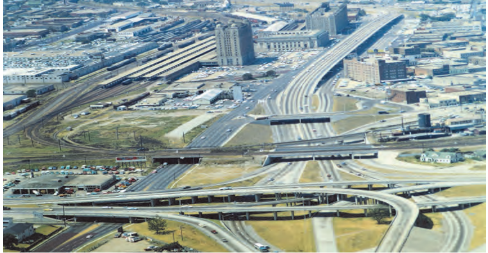
The U.S. 80/81 interchange was later redesignated the I-30/35W interchange in the early 1960s and named the Mixmaster for its overlapping and tightly curved ramps.
