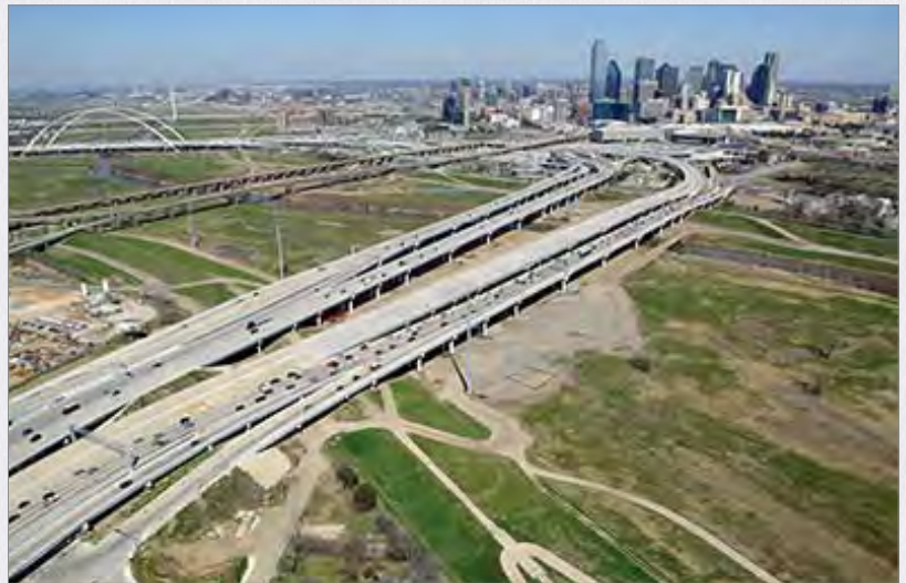
Pictured above: An aerial view looking north toward downtown Dallas at the bridge now carrying northbound I-35E traffic. This traffic switch occurred on March 25th.
