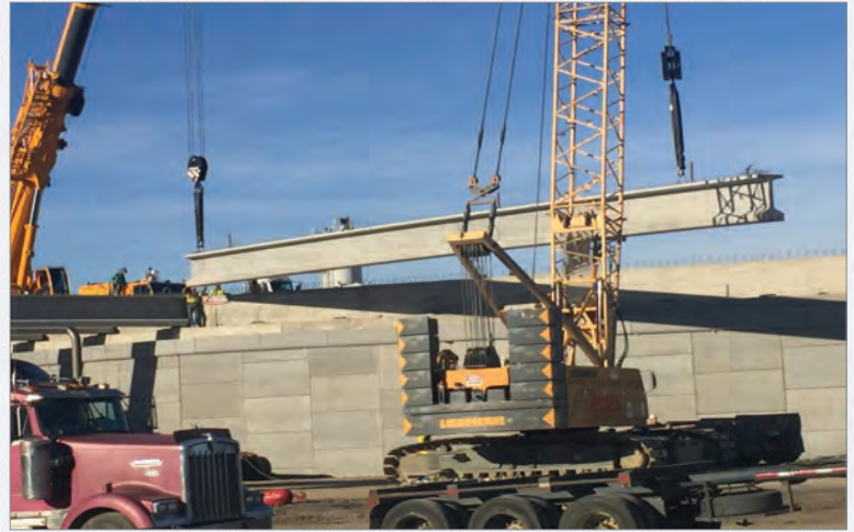
Crews set beams for the future SH 360 bridge at Heritage Parkway
