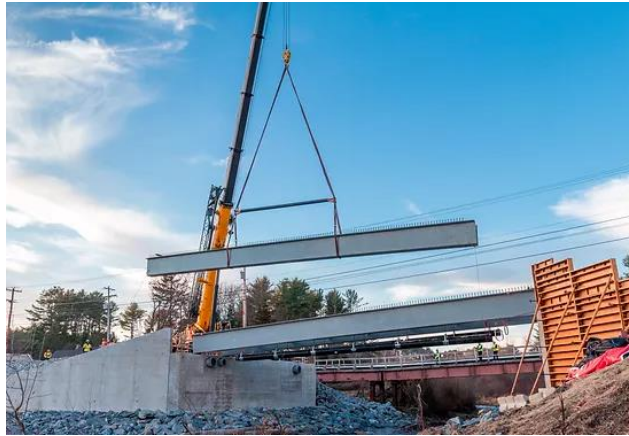
Figure 4.2.3-3 Construction of GBeam Bridge
