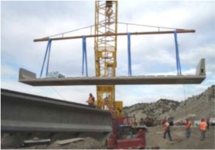
Figure G-10 - Transverse Slab Units with Attached Bridge Railing
