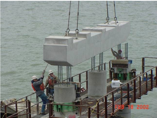
Figure G-11 - Installation of Precast Bridge Cap
