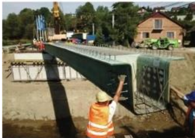
Figure 4.2.3-2 FRP Beam, Mostostal Warszawa
