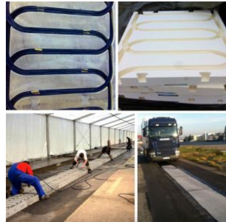
Figure 1.2.3-2 IPT PRIMOVE Dynamic Charging Installation in Mannheim, Germany
