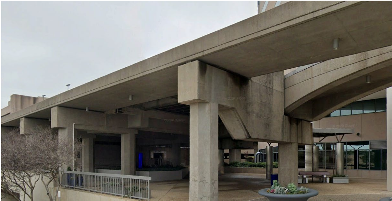
Figure 2-5 – Existing Area Under Potential Retrofit Roundabout
