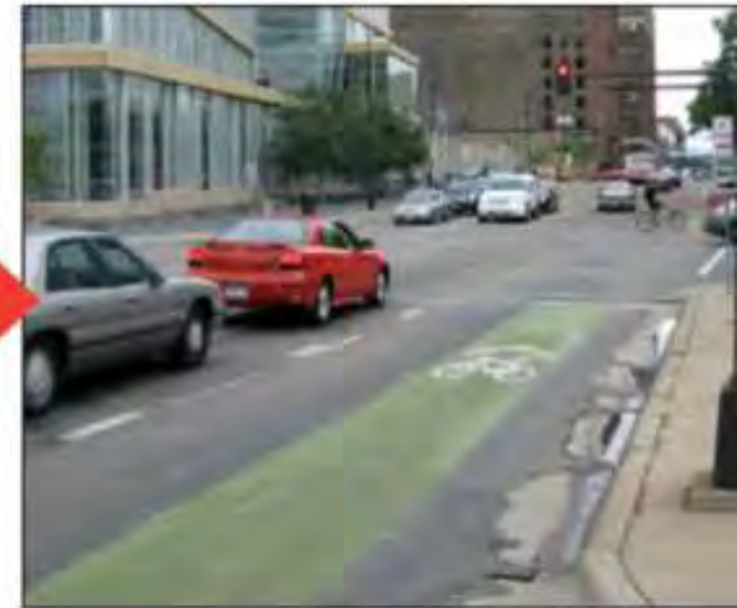
Green Shared Lane (Installed Summer 2010)
