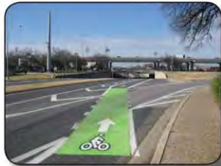
Figure 3-16 Example of a green bike lane being used at a conflict area where the bike lane crosses the right turn lane; Source: Halff Associates, Inc.
