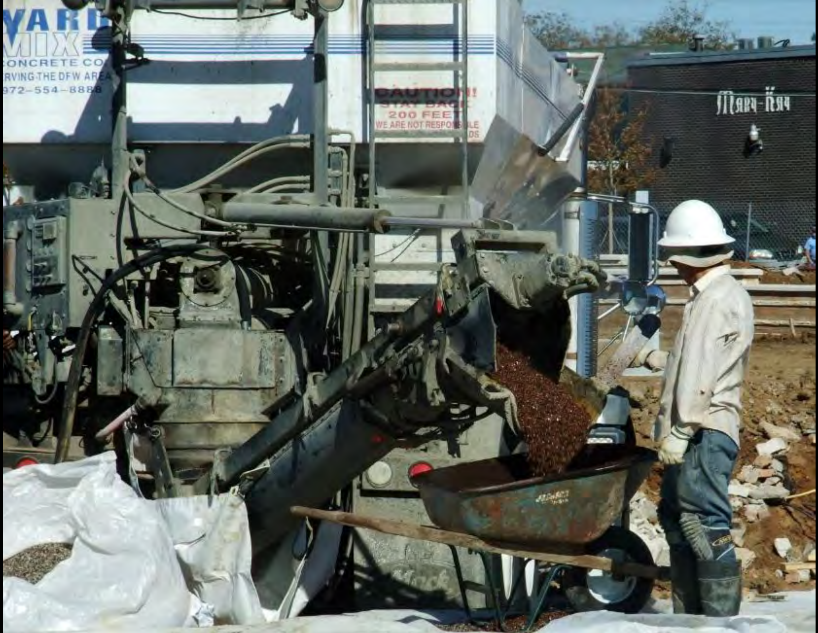
UTA Green at College Park: November 8, 2010: Filter Pave System
