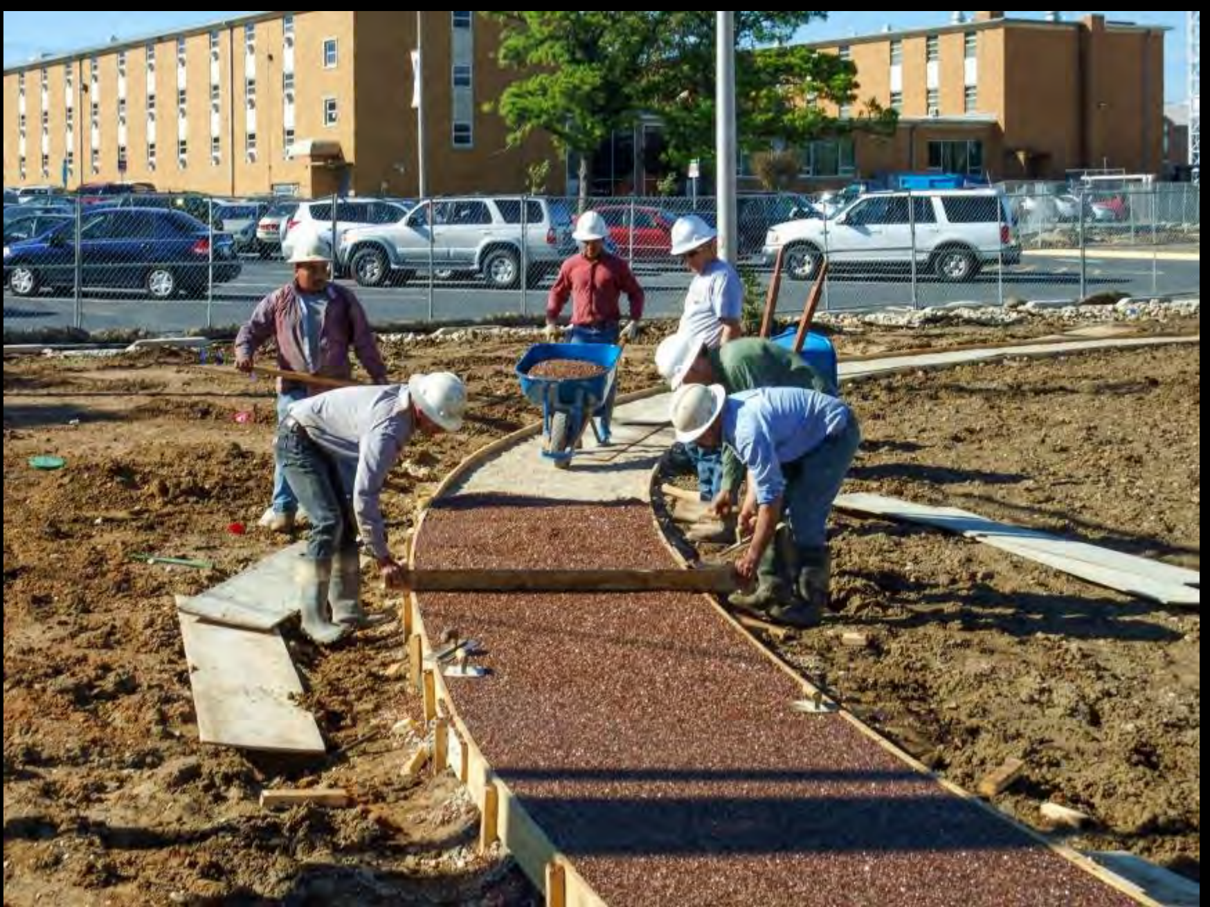
UTA Green at College Park: November 8, 2010: Filter Pave System
