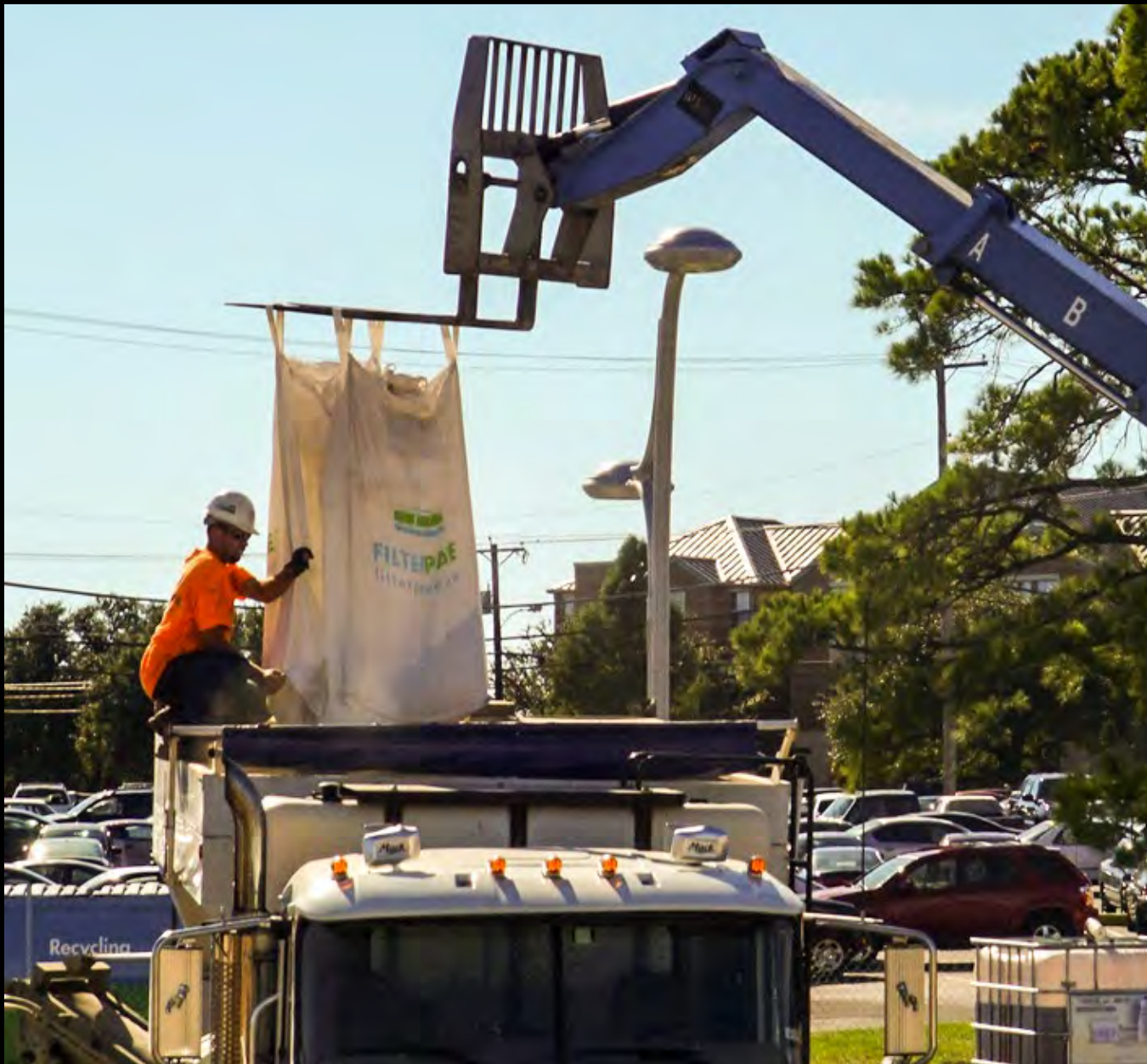
UTA Green at College Park: November 8, 2010: Filter Pave System
