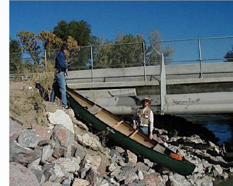
Poor Design: Steep slope, rugged terrain
