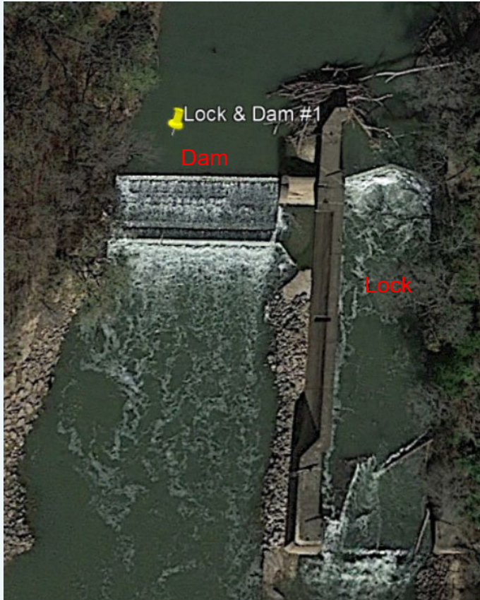
Lock & Dam #1 aerial view
