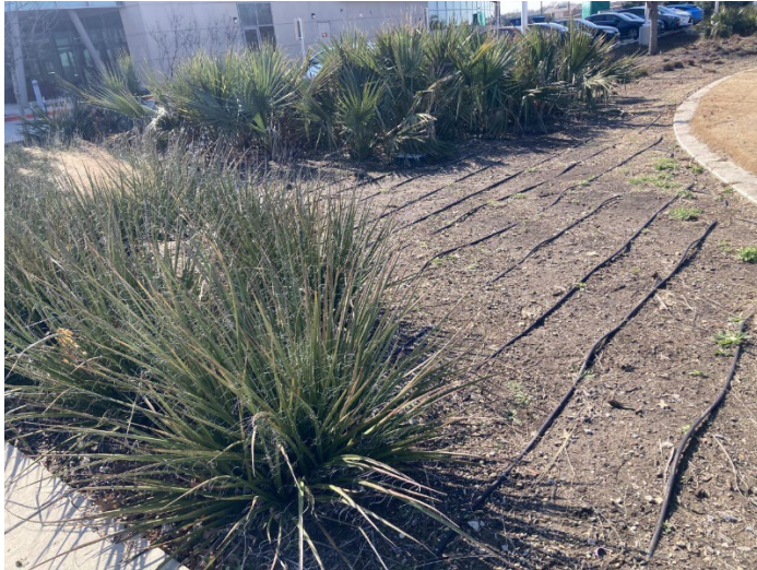
Figure 3. A bioretention area at a parking lot (Texas A&M AgriLife Extension Dallas Center, photo by Yufan Zhang)
