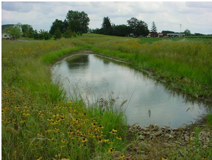
Figure 8. Wet detention pond (Minnesota stormwater manual, 2012)
