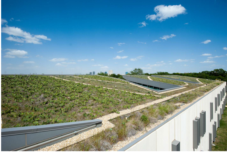
Figure 4. Green roof (Fort Worth Botanic Garden, n.d.)
