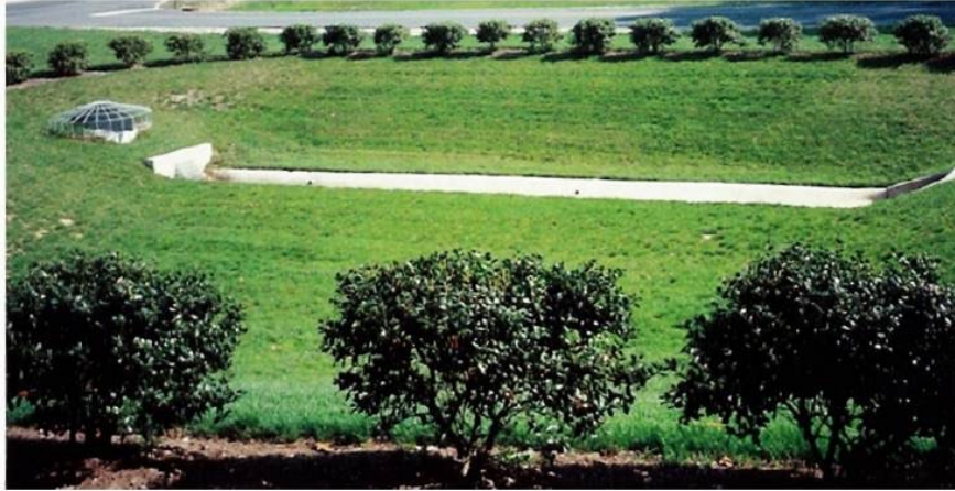
Figure 7. Dry detention pond (Minnesota stormwater manual, 2012)
