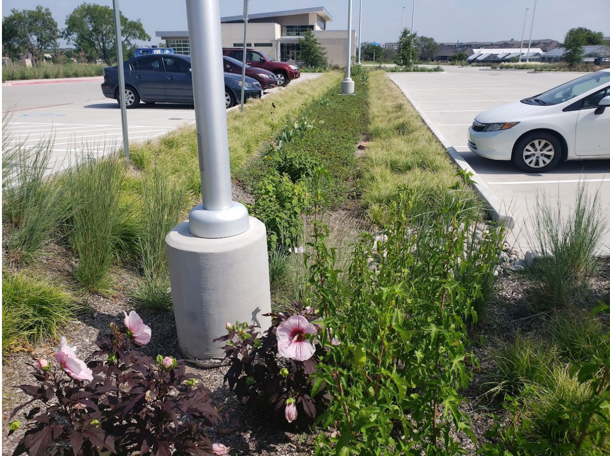
Figure 10. Bioswale at a parking lot (Texas A&M AgriLife Extension Dallas Center, photo by Fouad Jaber)
