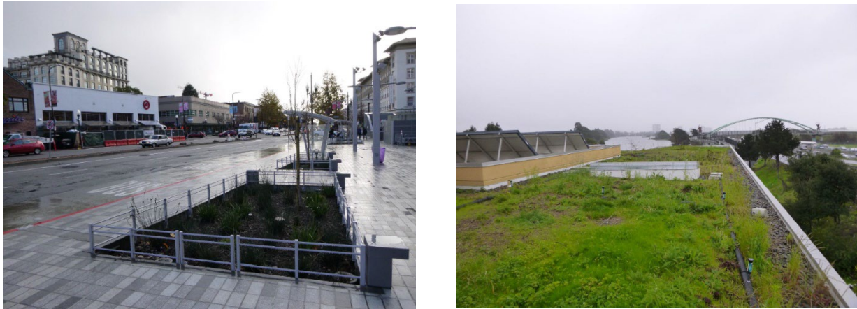
Figure 3. GSI applications in Berkeley (left to right, top to bottom: bioswales, permeable pavements, flow-through planters, green roofs)
