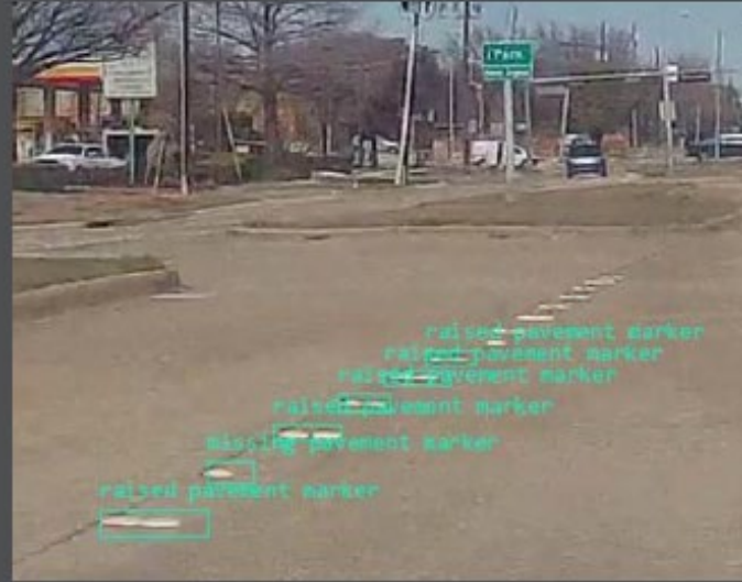
Figure 13. This figure shows show two different examples of missing raised pavement markings
