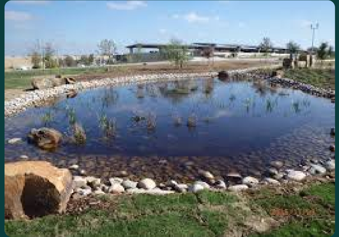
Detention Pond • TRWD Campus
