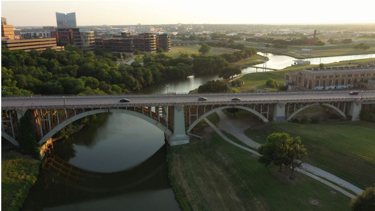
Cars drive across the Main Street Viaduct, which passes over the West Fork of the Trinity River north of downtown Fort Worth. (Rodger Mallison | Fort Worth Report)
