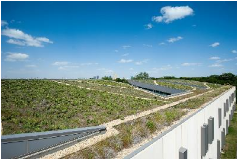
Green roof (Fort Worth Botanic Garden)
