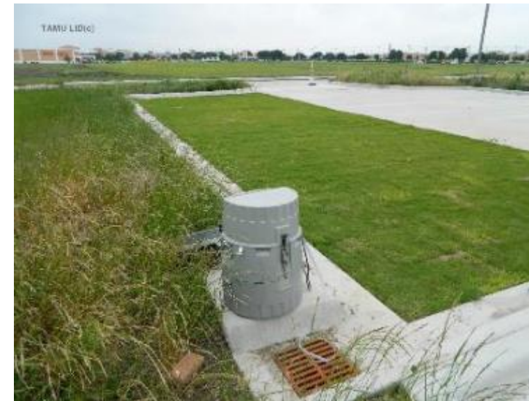
Permeable pavement (AgriLife)
