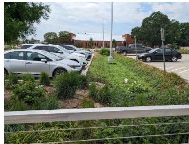
Bioswale/bioretention at a parking lot (AgriLife)
