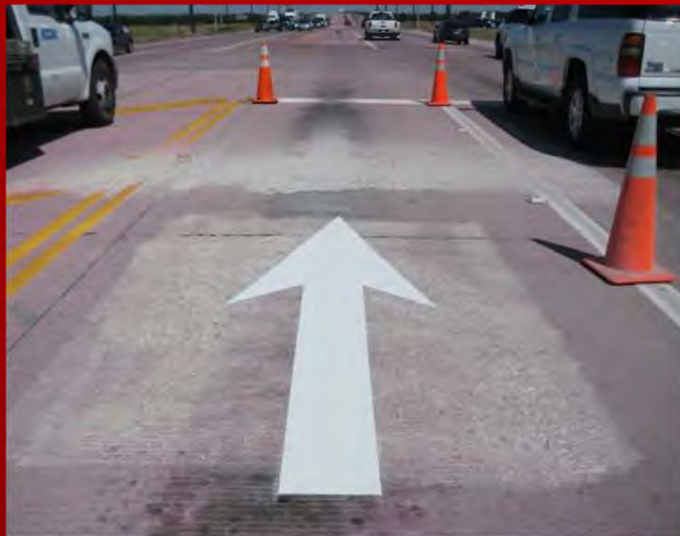
Modify Pavement Markings
