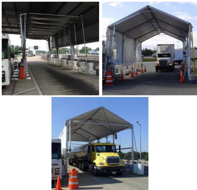
Figure 6: Previous OHMS Installations (2,3,4)
