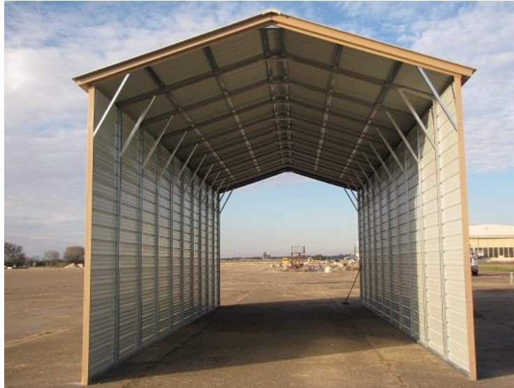
Figure 1: Shed Installed at the TAMU RELLIS Campus
