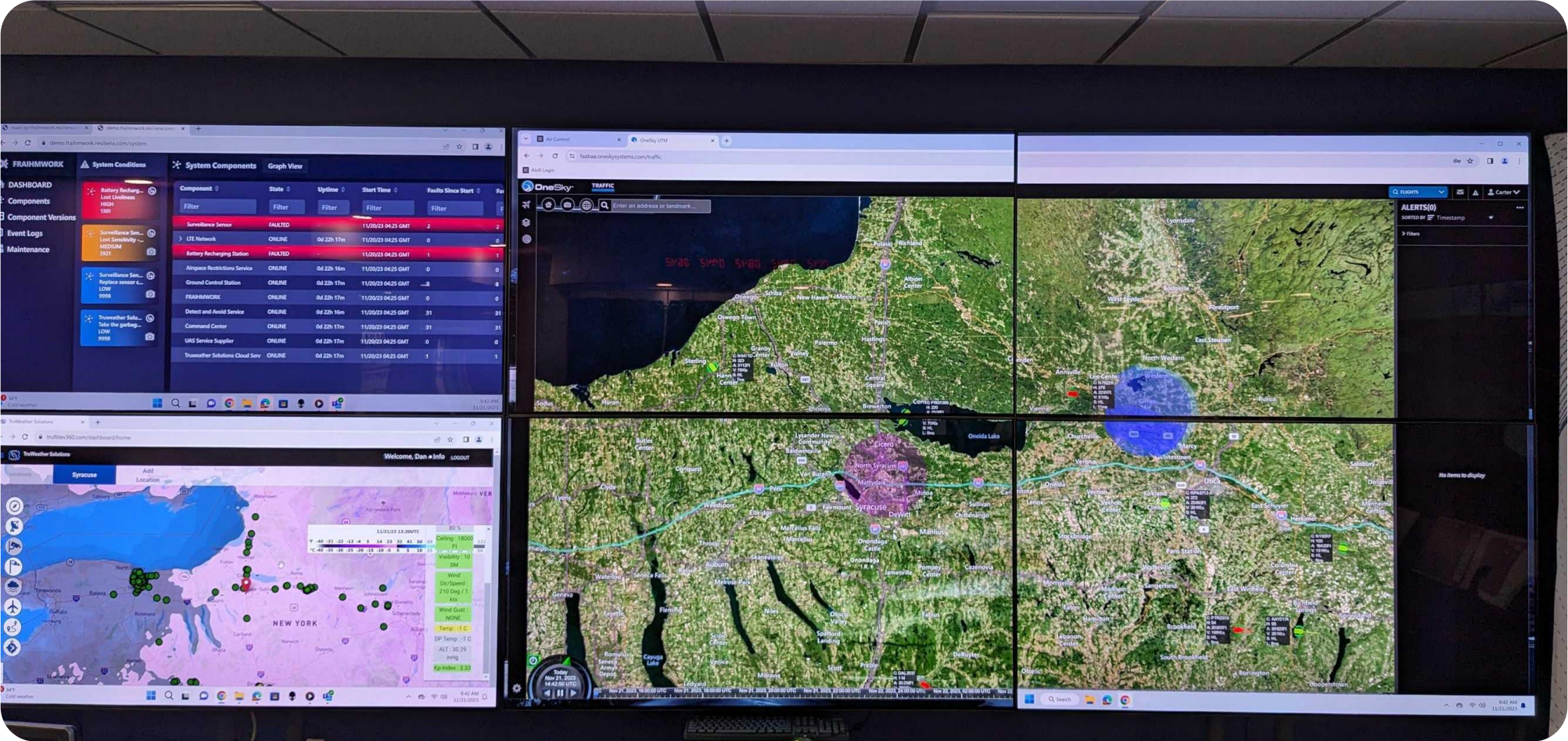
OptiX-GS Deployed at the Syracuse Hancock Airport Operations Center
