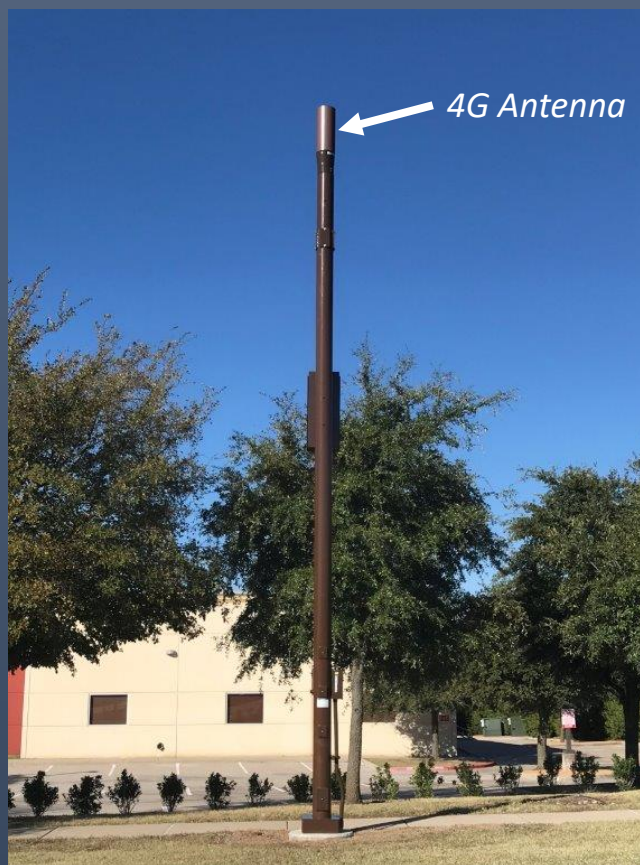
Node Pole Installation
