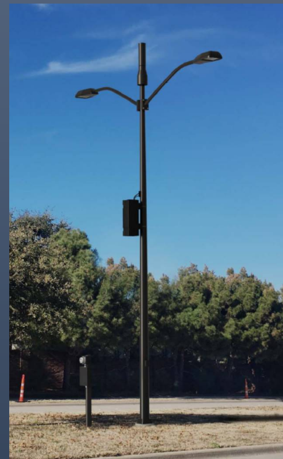
Service Pole Installation
