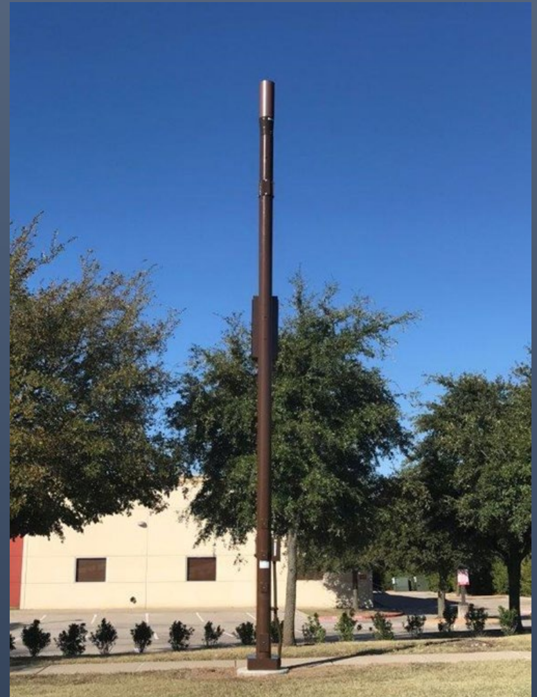
Node Pole Installation
