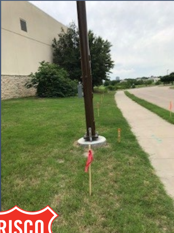
Installed on ROW line
