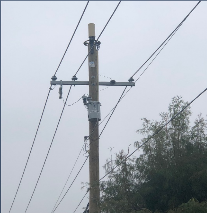
Utility Pole Installation
