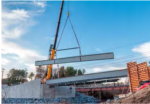
Figure 4.2.3-3 Construction of GBeam Bridge
