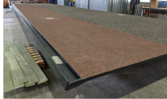
Figure 6.1.2-3 Polymer Panel for Potential Retrofit Deck
