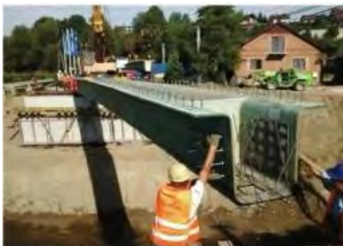
Figure 4.2.3-2 FRP Beam, Mostostal Warszawa
