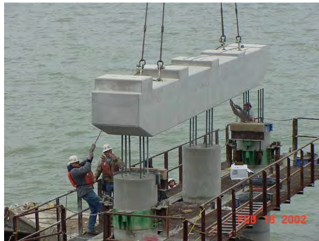
Figure G-11 - Installation of Precast Bridge Cap
