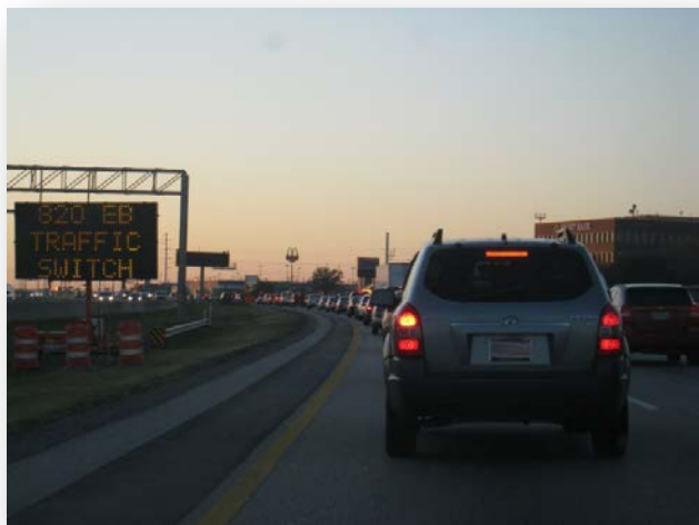
IH 820 Construction North Richland Hills
