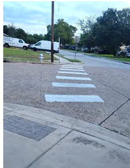
The curb ramp is not in line with the crosswalk.
