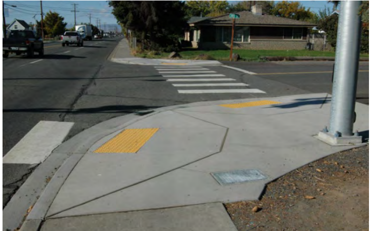
Example of ADA curb ramps that follow best practices of aligning with the center of each crosswalk.
