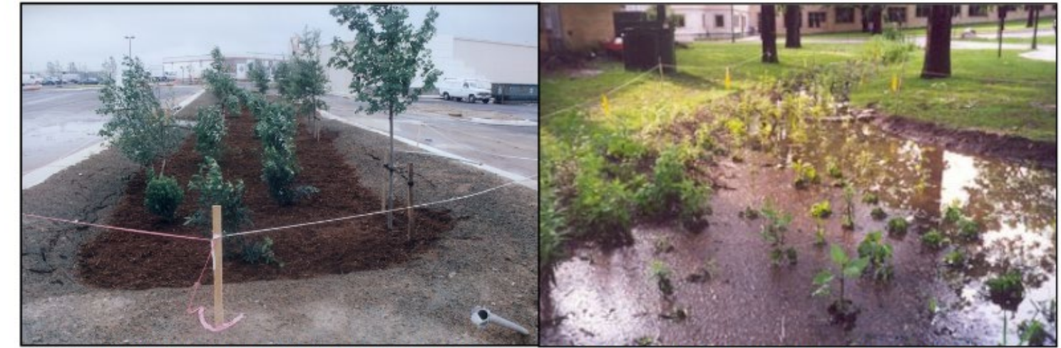
Newly Constructed Bioretention Area
