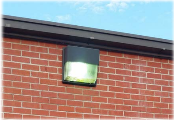
Malfunctioning Photocells
