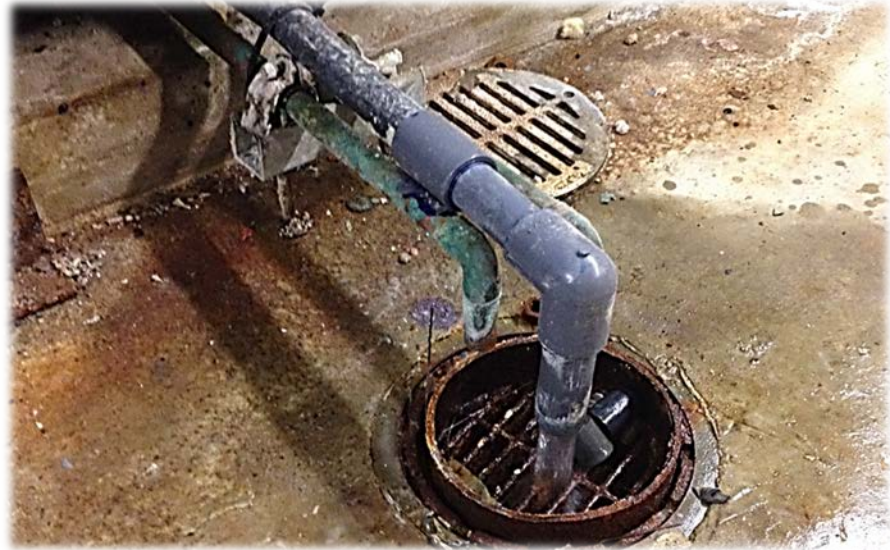
Cooling Tower Blowing Down
