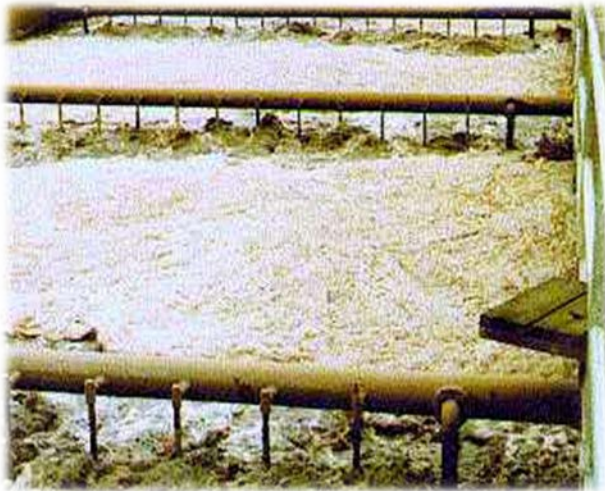
Coarse Bubble Aeration
