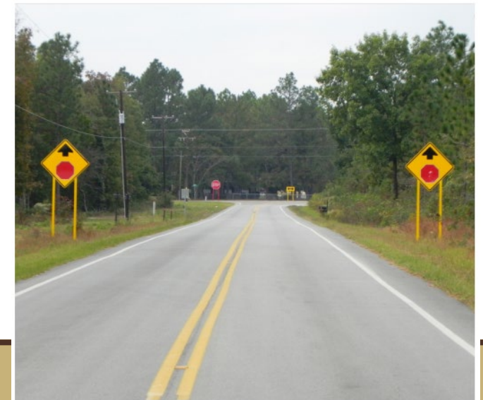
Example of countermeasures on the stop approach. Source: South Carolina DOT
