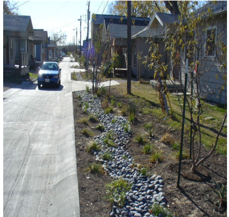
Bioswale and landscaping
