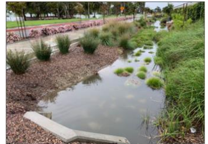
A bioswale along the side of a roadway in Orange County
