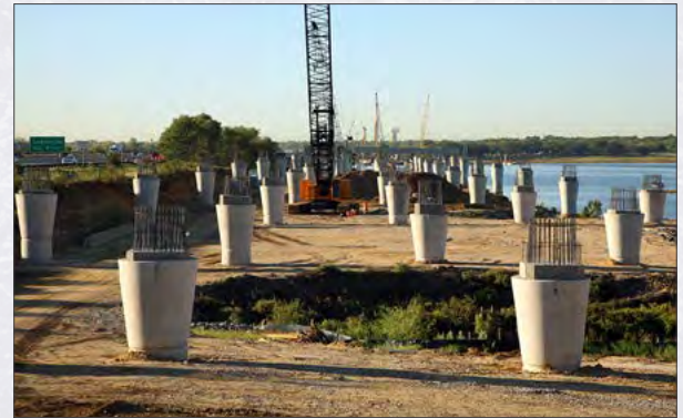
Column construction and beam placement for the new southbound Lewisville Lake Bridge (looking south towards Lewisville)
