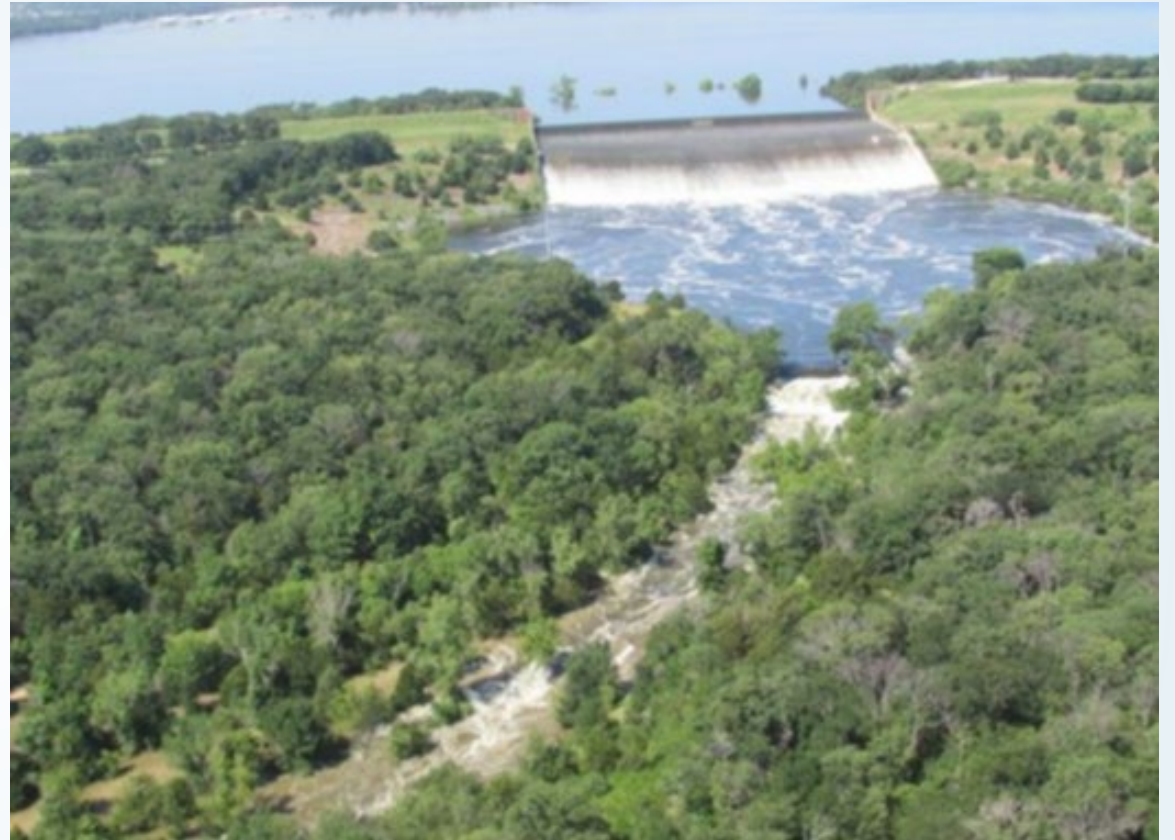
H. Grapevine Lake Spillway, June 19, 2015
