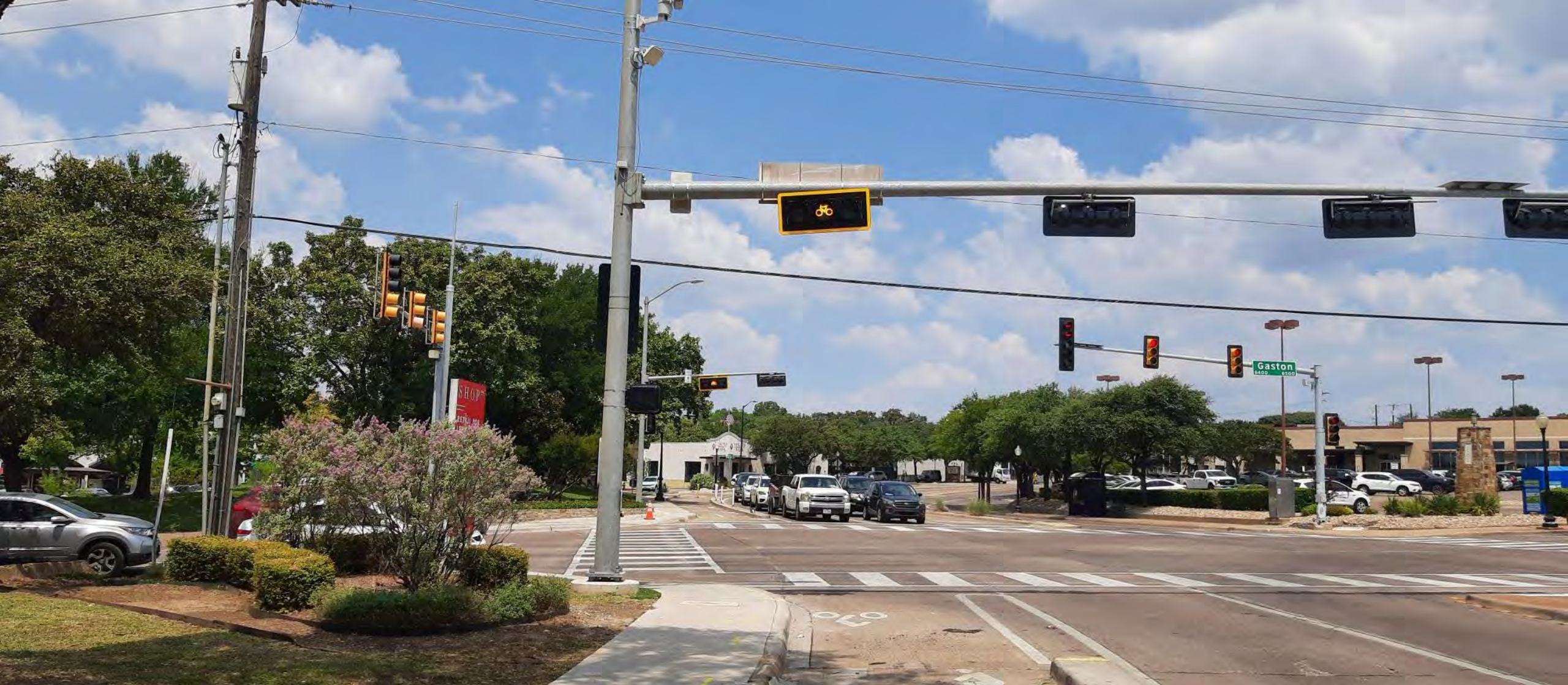
Abrams at Gaston: Northbound view
