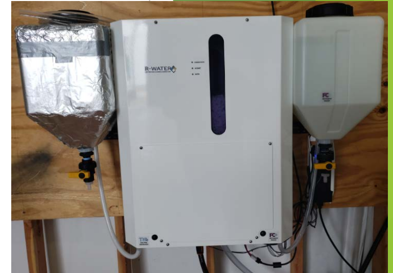
R-Water Unit makes on-demand hypochlorous acid
