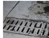
Do not let water from washing, discharge points, oil traps, filters and separators run to stormwater drains.
