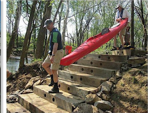
Good Design: Wide, sturdy staircase
