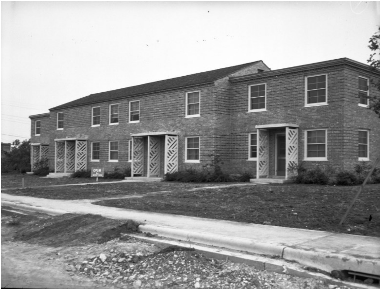
Exterior view of Butler Place, a government housing project built in the 1940s for African American residents in the Chambers Hill district of Fort Worth. A sign in the front yard reads, "Open for Inspection." (Courtesy photo | UTA Libraries Digital Gallery)
