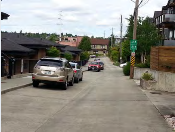
New Urbanist Skinny Street with Center of Street Drainage
