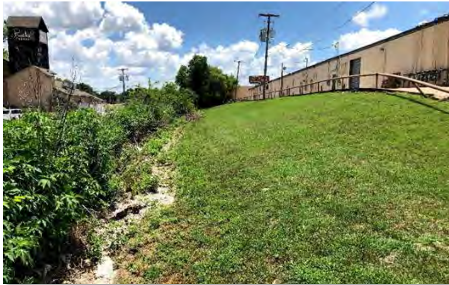
Figure 22 – Existing Drainage Channel
