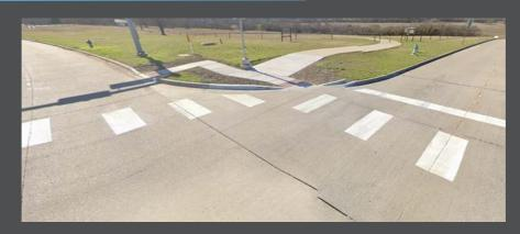
Figure 3. Los Rios Boulevard and Parker Road- The City of Plano Transportation Division identified crosswalk pavement markings that were not aligned with the pedestrian ramp in the northwest corner.
