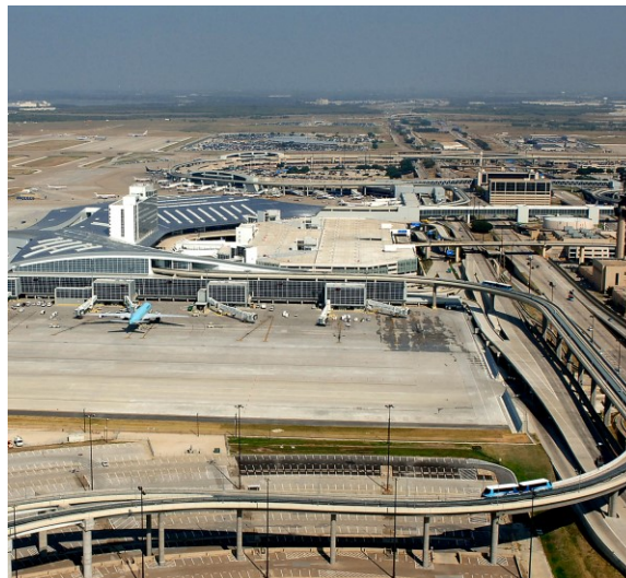
Figure 1: Dallas/Fort Worth International Airport's Skylink people mover system uses rubber-tired vehicles traveling on a double-tracked elevated guideway to connect the airport's passenger terminals. 7
