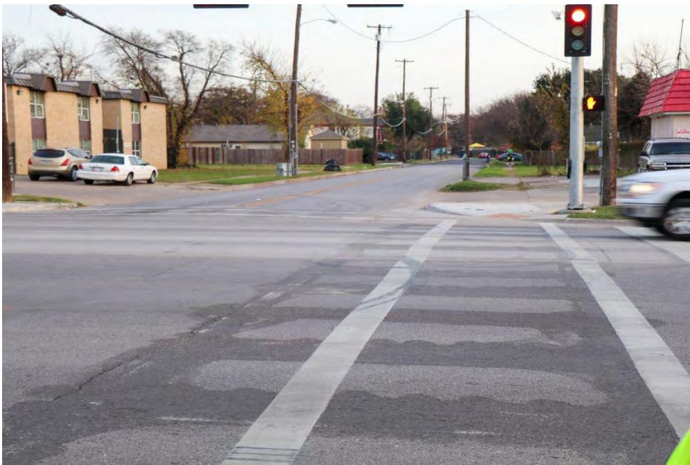
Figure 19: Crosswalk at Holmes, showing removed ladder style markings, and tire marks from cars doing "donuts."
