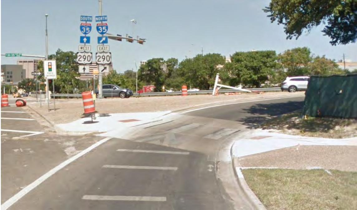
Figure 4: Example of a raised crosswalk on a turn lane joining an interstate frontage road in Austin, TX. (Source: Google Street View <https://goo.gl/maps/PnLAq25X2tKVjf8e9> )
