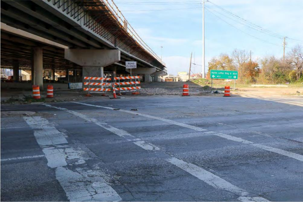
Figure 11: Stop bar and crosswalk markings that should be removed as they are no longer applicable.
