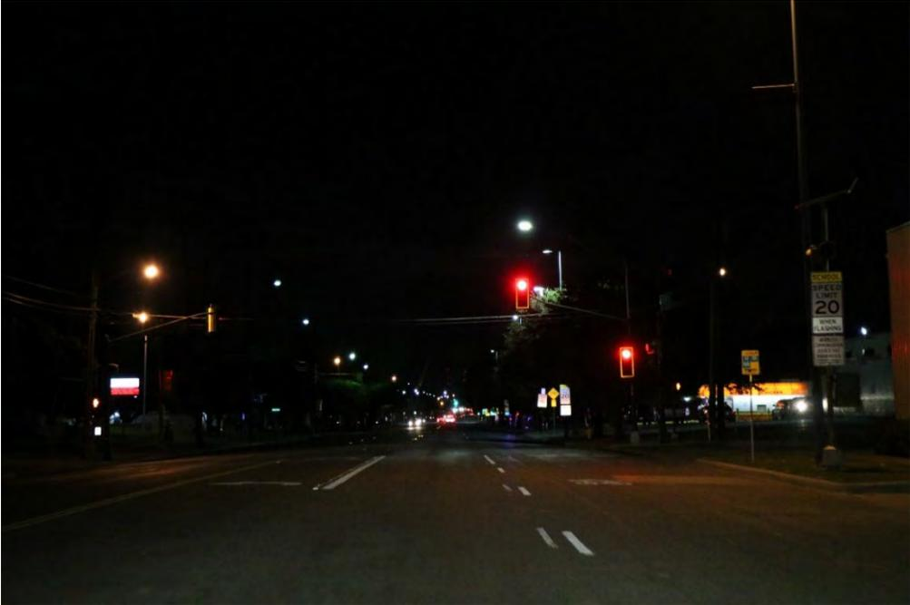
Figure 5: Meadow intersection at night, with missing street name sign on the westbound approach. The addition of the retroreflective background around the signal helps with visibility of the signal indications.
