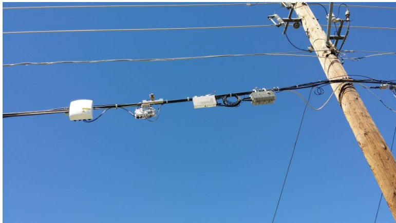
Strand mounted equipment and antenna
