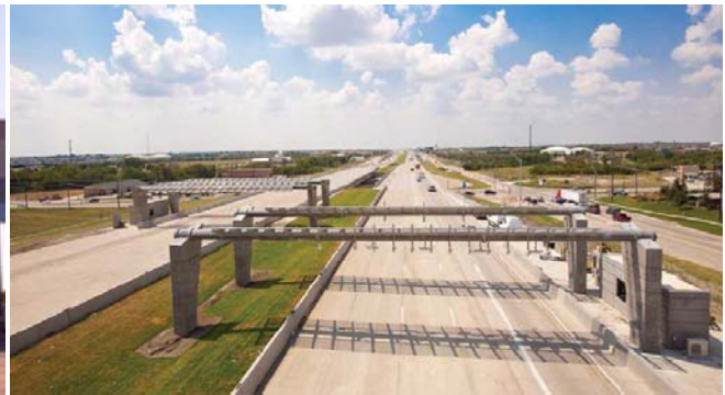
SH 190 Toll Plaza (NTTA.ORG)
