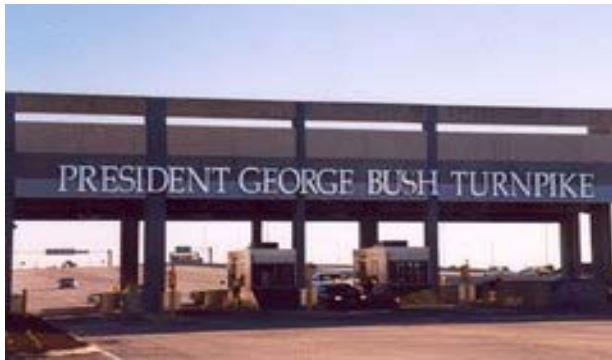
PGBT Eastern Extension Toll Plaza (NTTA.ORG)
