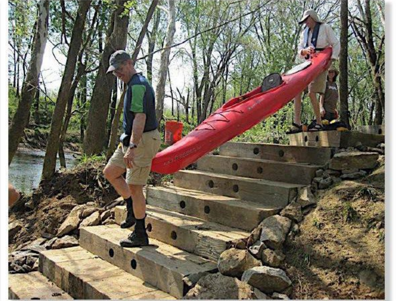
Good Design: Wide, sturdy staircase
