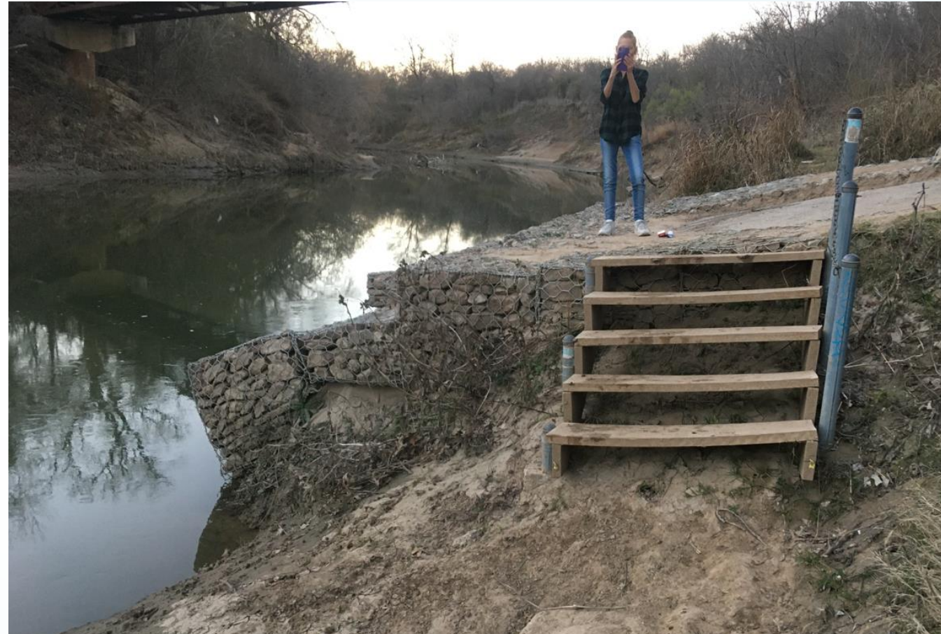
Launch does not go completely down to the water. The steps lead to the water level for a temporary launch from the bank.
