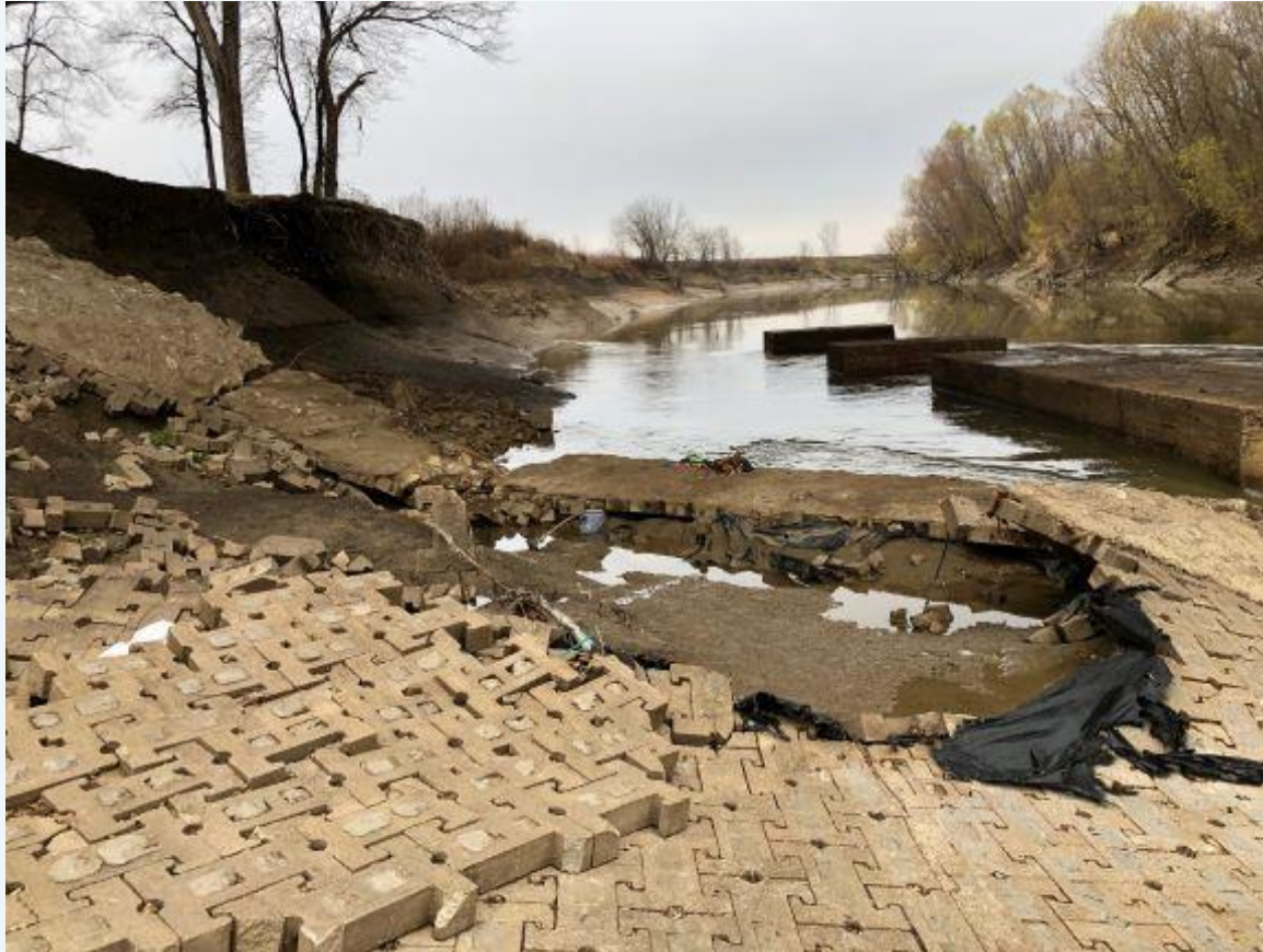
Loop 12 Boat Ramp Upstream side
