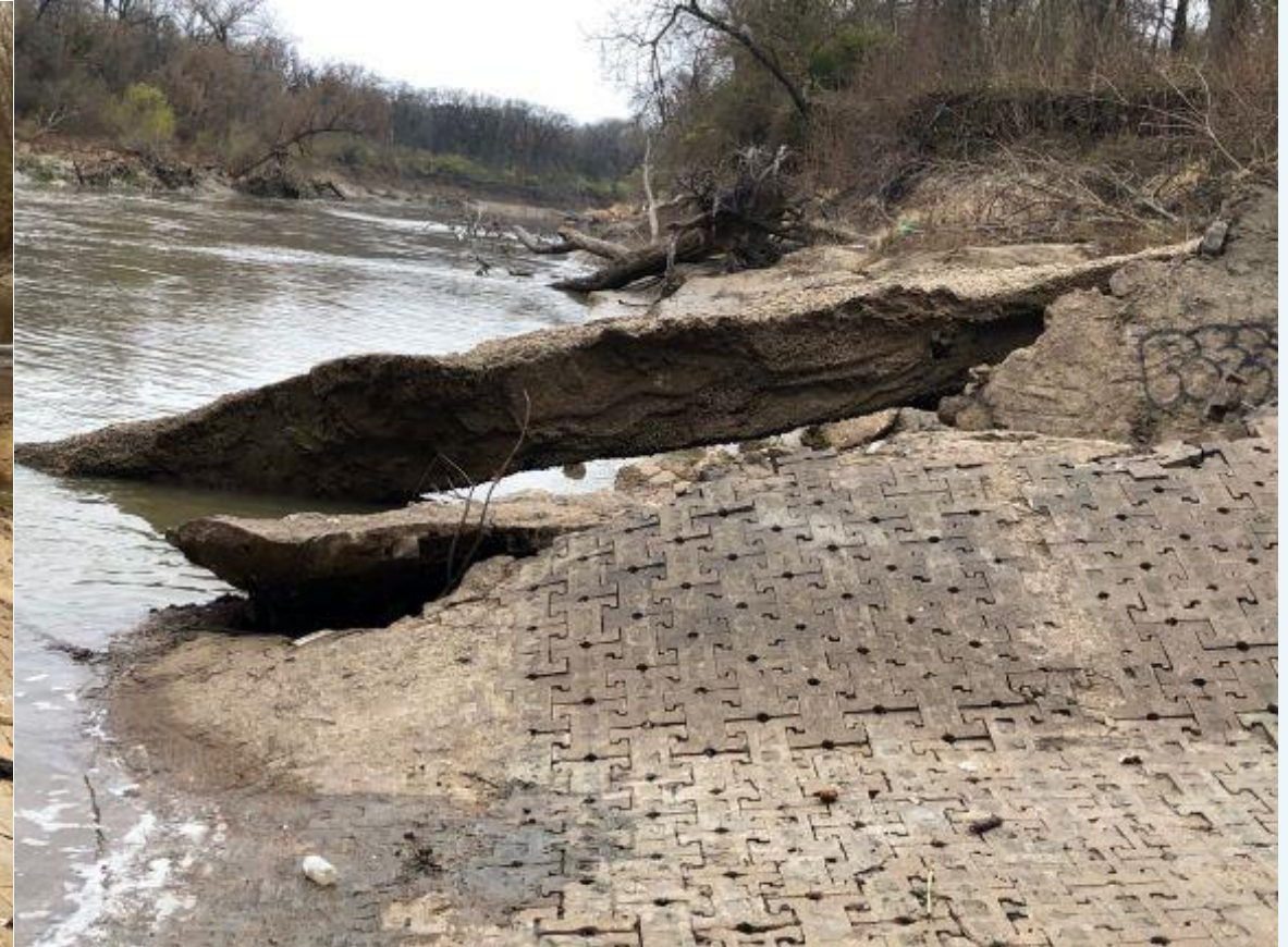
Loop 12 Park Boat Ramp Downstream side
