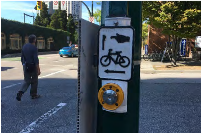
A dedicated bicycle signal actuated by a push button at the intersection.
