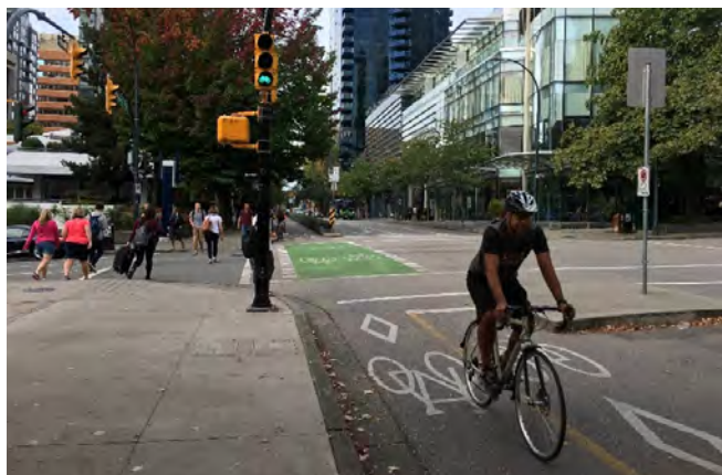
A median island can provide safe refuge for bicyclists travelling across an intersection.
