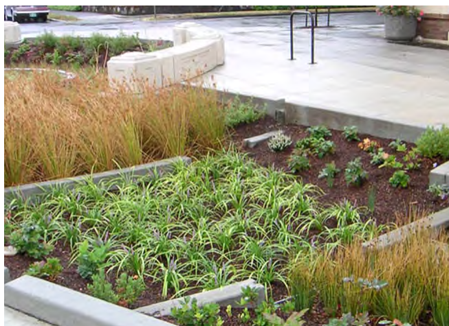
Green infrastructure may include rain gardens or bioswales, which absorb stormwater runoff and can be placed within curb extensions or islands.
