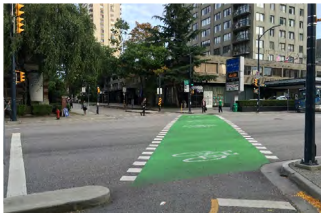
Green pavement markings are used to identify where bike facilities transition through an offset intersection.
