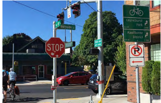
Pedestrian Hybrid Beacon (HAWK) signals may be used for bicycle intersection crossings where a full traffic signal is not warranted.
