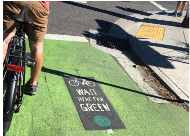
Bicycle detection installed at an intersection may be used in addition to activating a push button.
