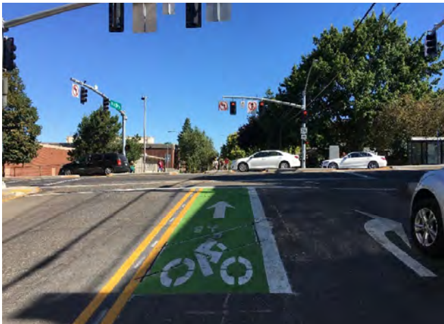
Example of a bicycle detection with a bicycle signal phase installed at a bicycle boulevard intersection of a major roadway.
