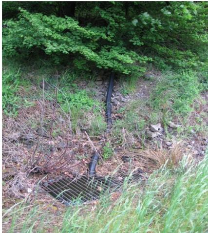
A surface hose discharging into a storm drain inlet. This may be an illicit connection. (photo courtesy WSDOT)
