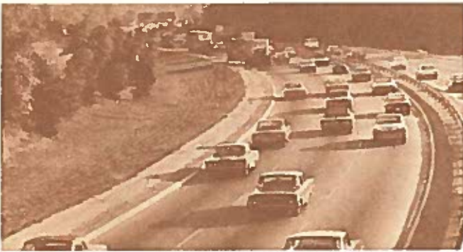
Level of Service C: Stable flow of traffic, but drivers having restricted freedom to select their own speed, change lanes, or pass.
